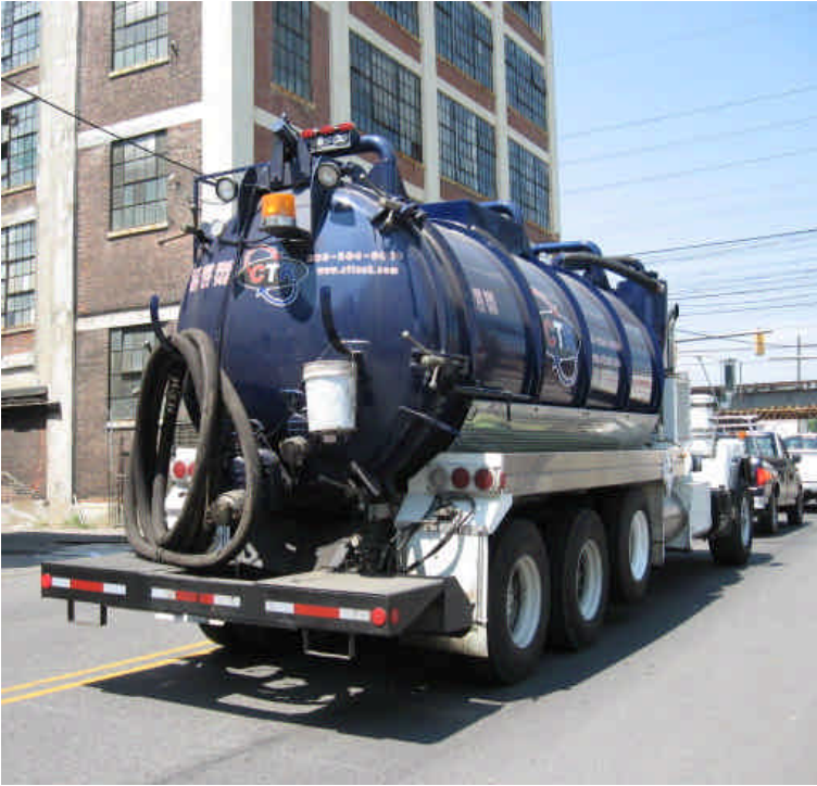
Vac truck returning to the site for dewatering the excavation
