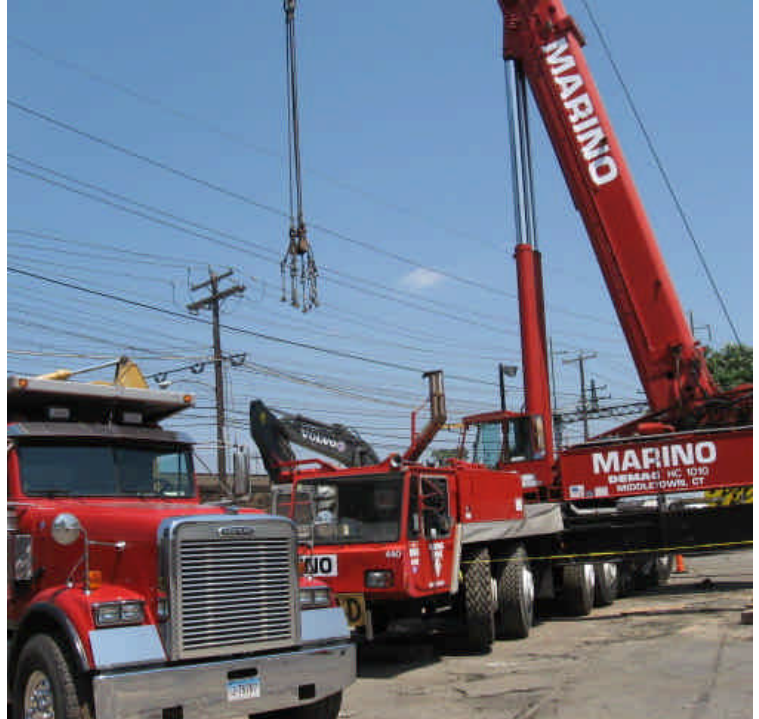
Overview of equipment in place for the vault construction.
