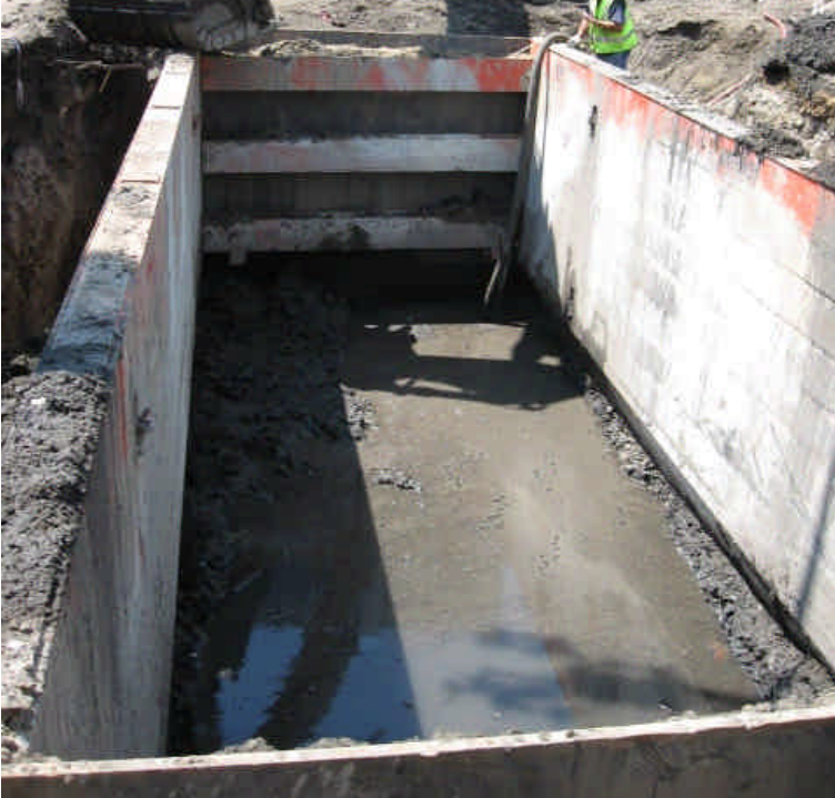
Open trench being dewatered and prepared for vault installation.
