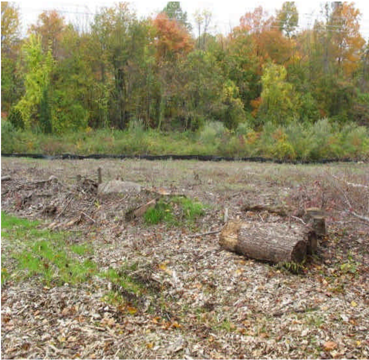
Silt fence off High Hill Rd.
