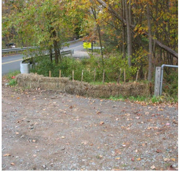
Extra haybales added to prevent runoff at Mansion Rd. entrance.
