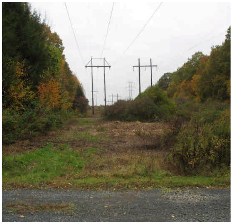
Vegetation left in place for stabilization off Old Farm Rd.
