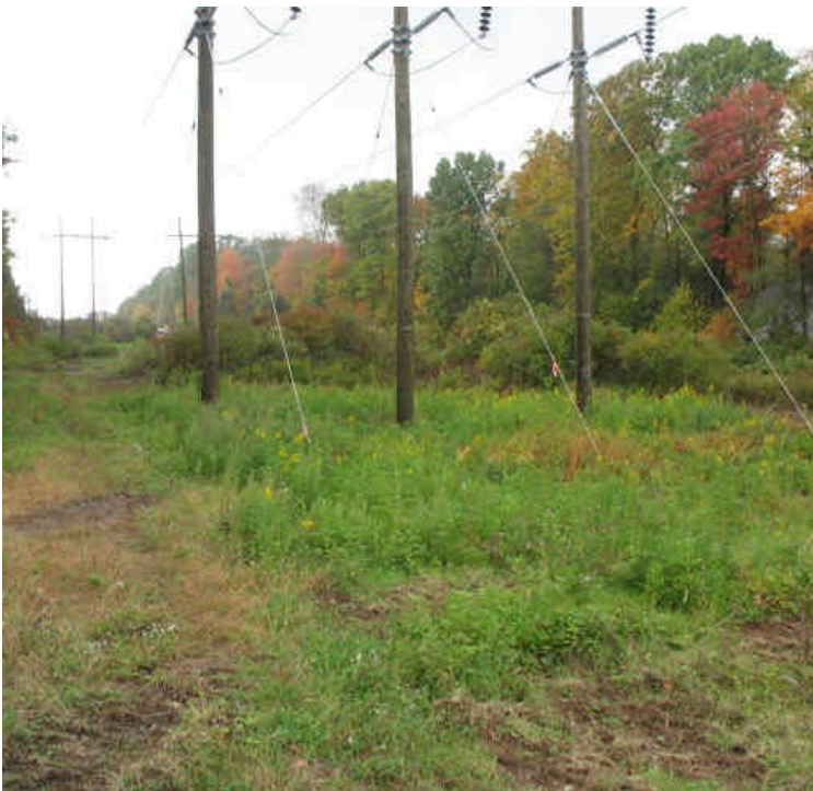
Shrubs left in place to stabilize slope off Old Farm Rd.
