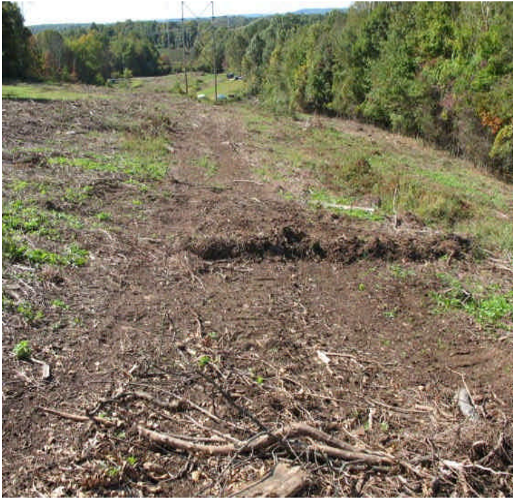
Water bars located on the skidder path off High Hill Rd.
