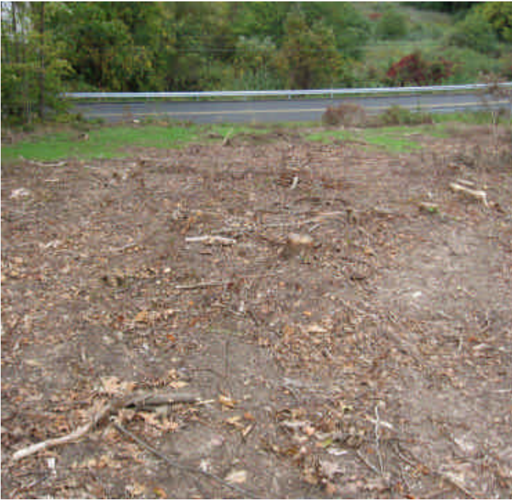
Roots left in place with grass growth downgradient on Mansion Road.
