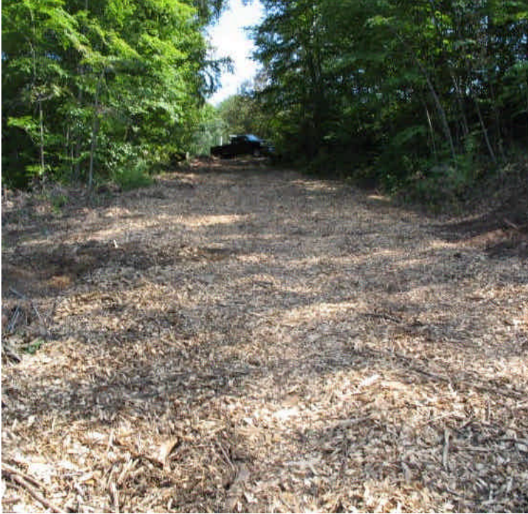
Entrance off High Hill Rd. Wood chips were placed to stabilize.
