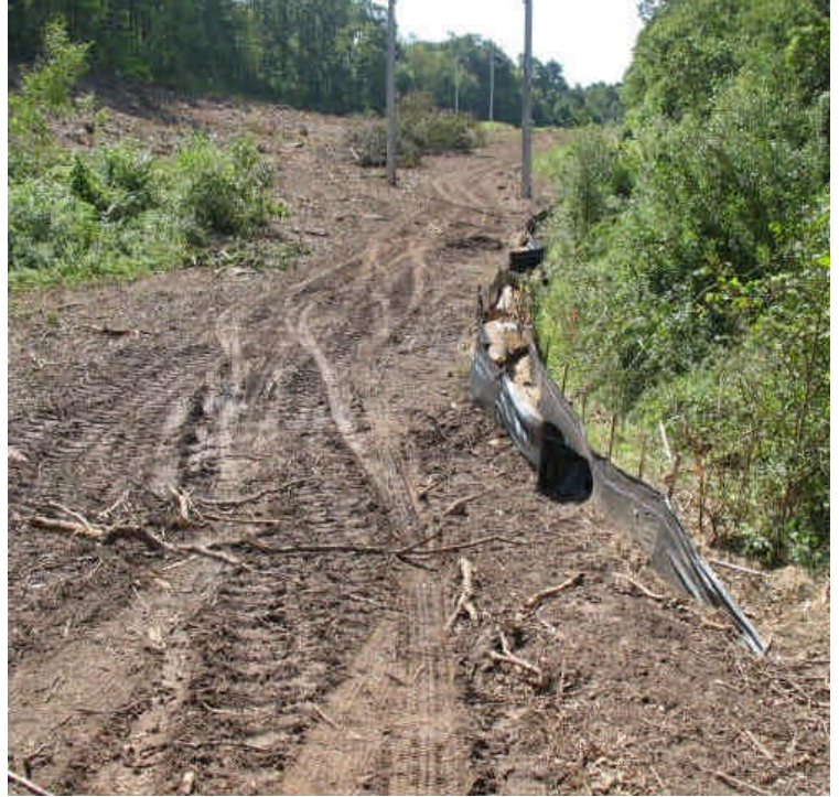
Erosion and sediment controls adjacent to the southern wetland at High Hill Rd.
