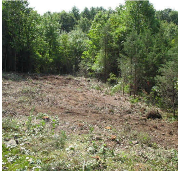
Right-of-way cleared, with vegetation left for erosion control, and 100' buffer maintained off South Turnpike.
