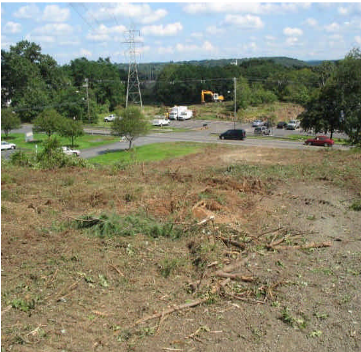
Recently seeded slope looking north over South Turnpike.
