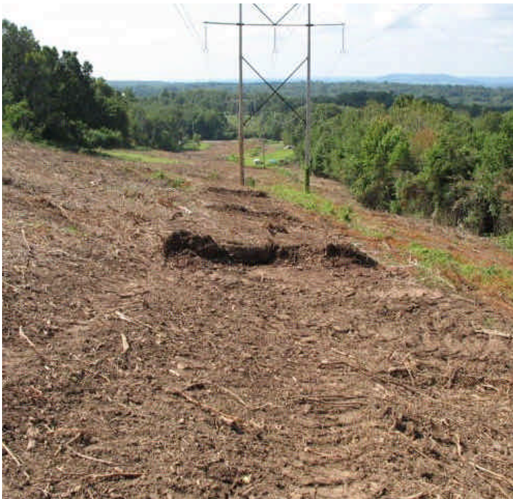
Water bars added between High Hill Rd. and Rt. 68.
