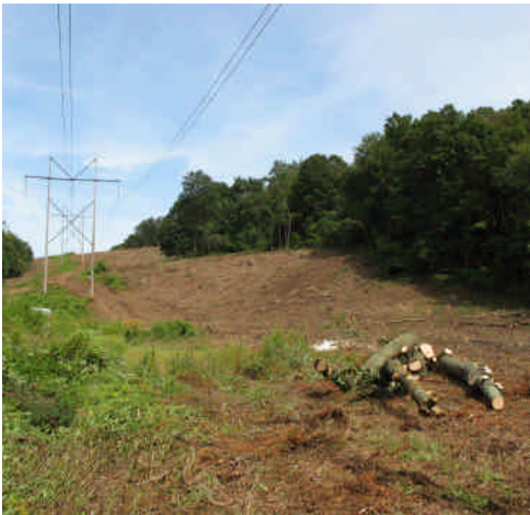
Exposed slope needs water bars and/or other erosion controls.
