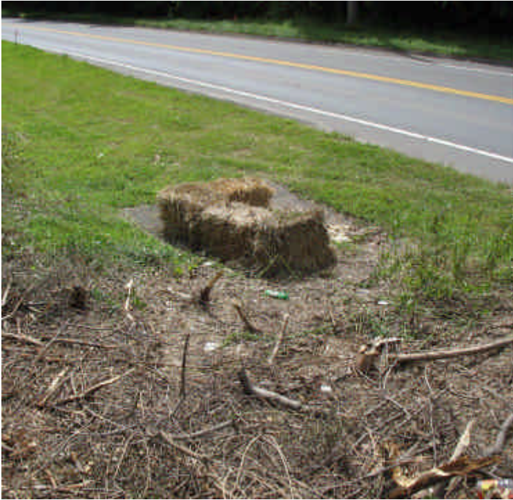
Haybales were installed off Rt. 68 at catch basin inlet.
