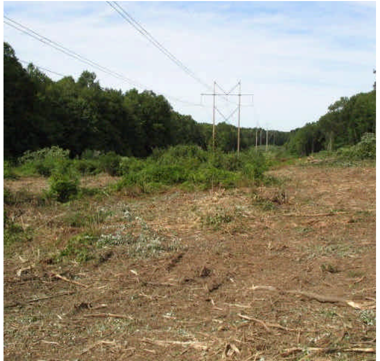
Right-of-way cleared, with vegetation/woody debris left for erosion control.
