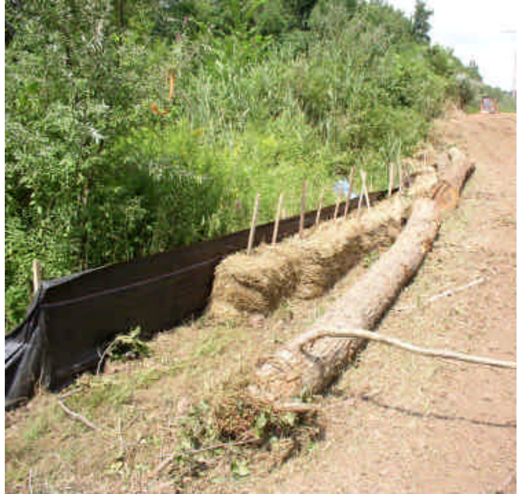
Erosion and sediment controls adjacent to the southern wetland.
