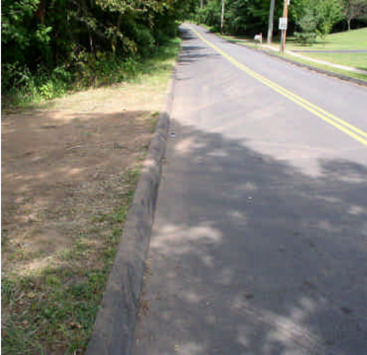
High Hill Road entrance to the ROW. Minimal tracking was noted.
