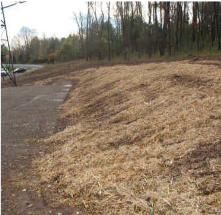
Mulch applied to most disturbed slopes off Route 66 (Black Pond).
