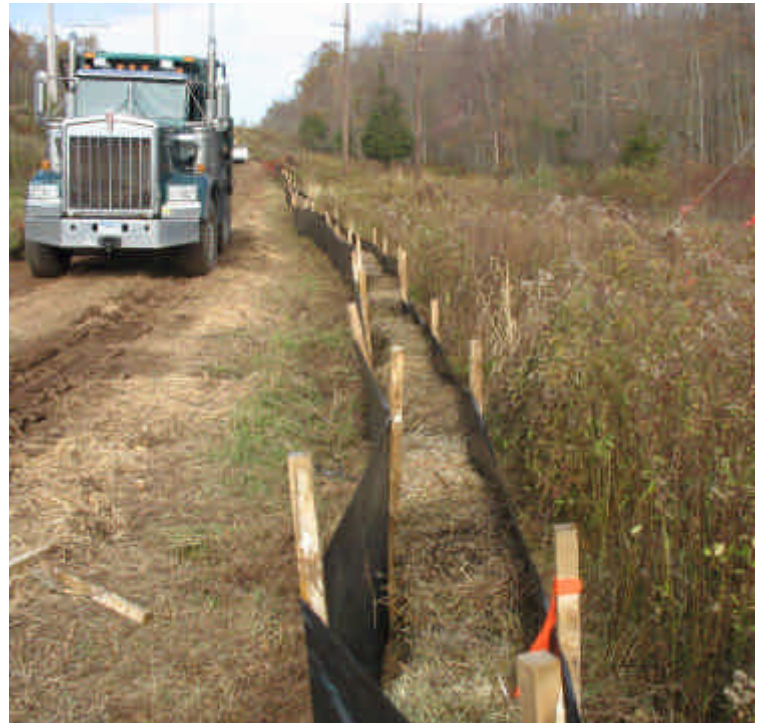
Silt fence/haybale barrier along the access road adjacent to the wetland near Beseck SS.
