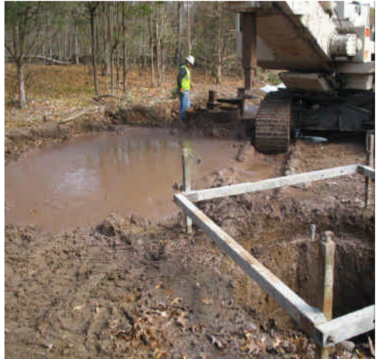
Slurry area from foundation drilling dewatering off Black Walnut Dr.
