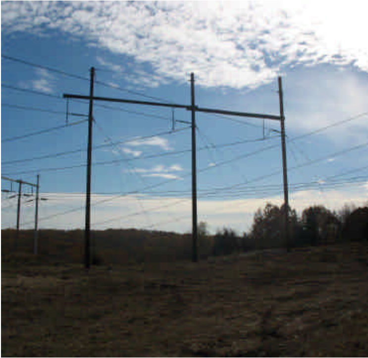
Pole installation complete at Oxbow Junction.
