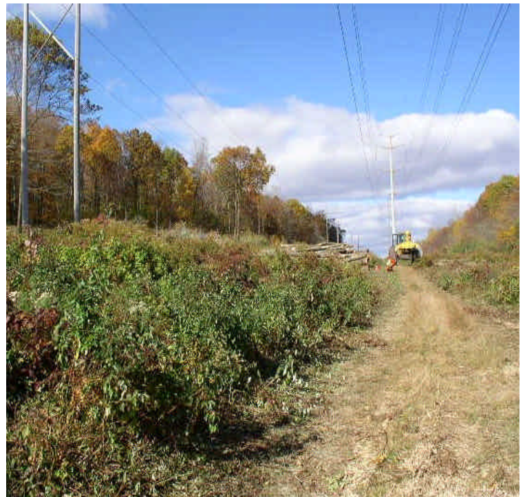
Tree clearing in the ROW, north of Beseck Switching Station.
