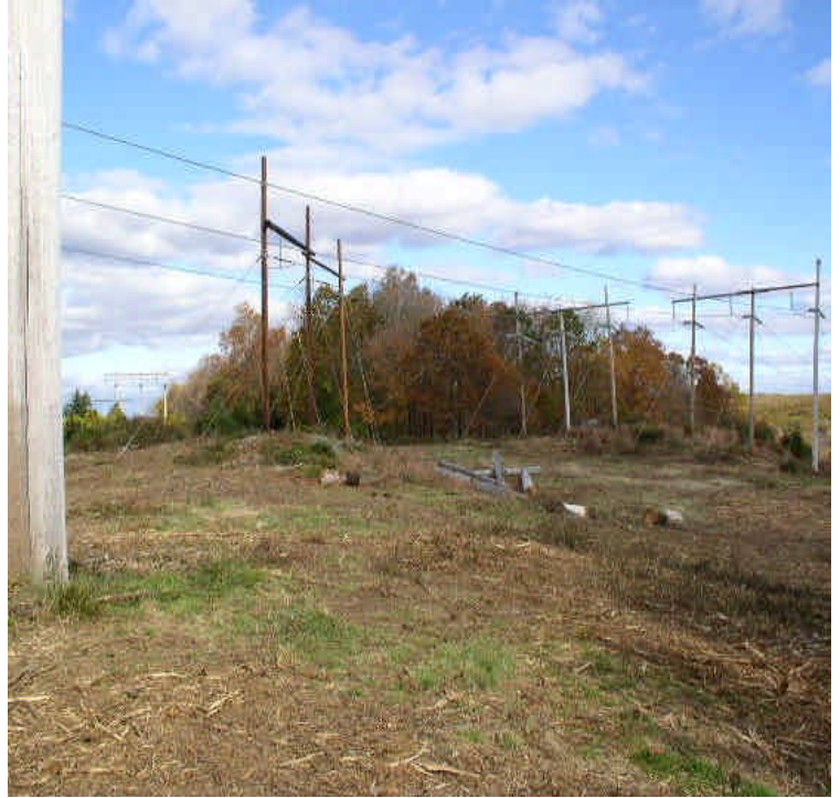
Pole installation complete at Oxbow Junction.
