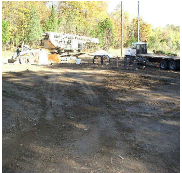
Drilling foundations off Black Walnut Dr.
