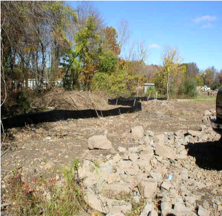
Silt fence installed at the contractor receiving yard & staging area.
