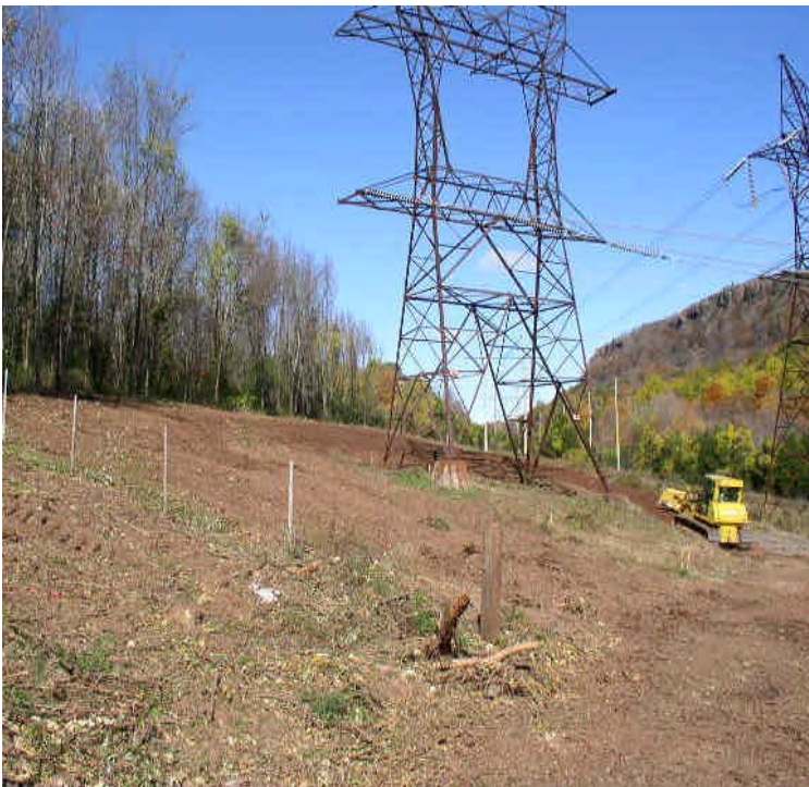
Grading and site preparation off Route 66 (Black Pond).
