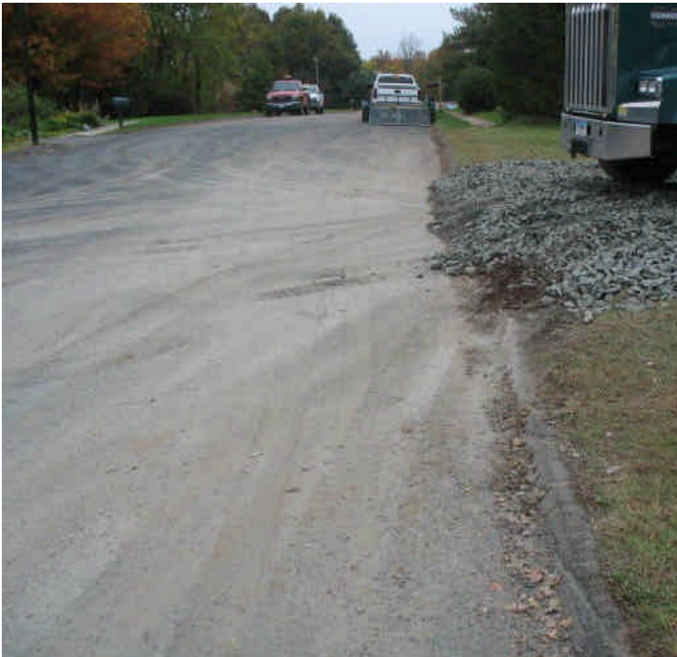
Minor sediment tracking onto roadway at Black Walnut Dr.
