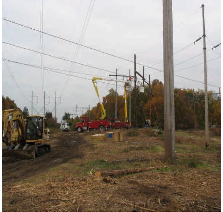
Pole installation at Oxbow Junction.
