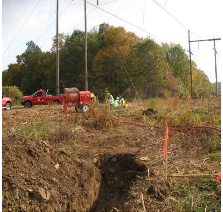
Foundation drilling and inspection at Oxbow Junction.
