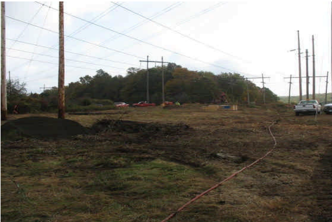
Vegetation clearing limits at Oxbow Junction. Foundation drilling underway.
