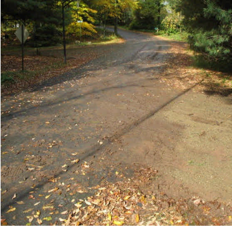
Mud and sediment tracking observed on Oxbow Road.
