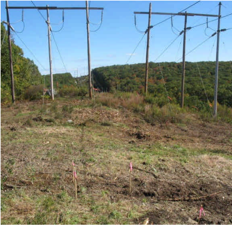
Vegetation clearing at Oxbow Junction.
