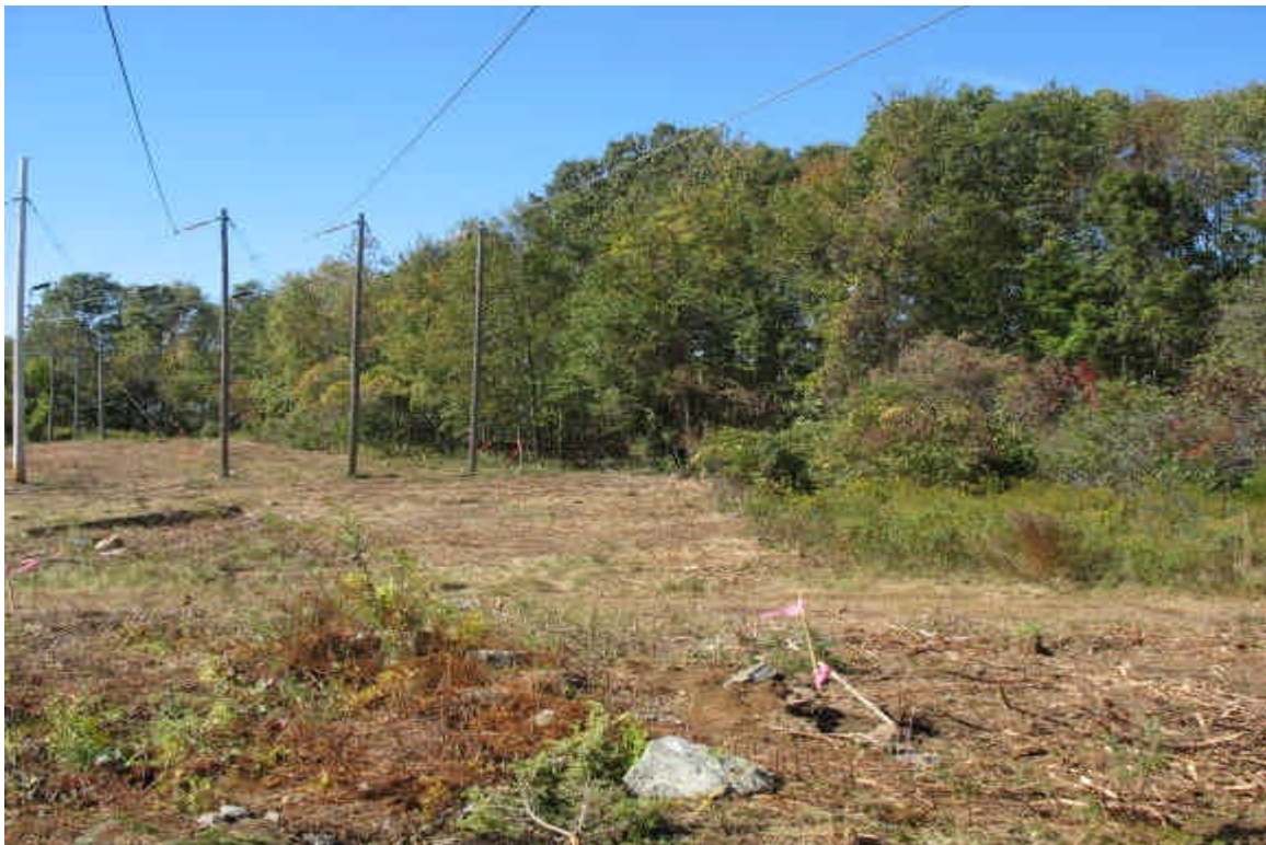
Vegetation clearing limits at Oxbow Junction. Archeological investigation is the only work occurring on site at this time.
