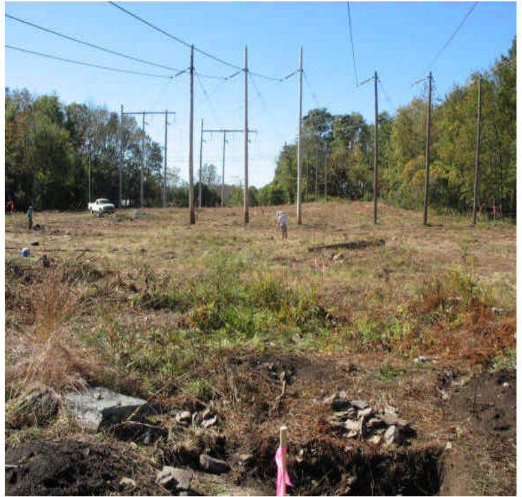
Oxbow Junction, looking west towards Beseck Switching Station.
