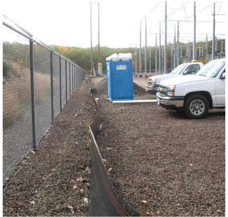
Silt fence along the eastern perimeter fence looks good.
