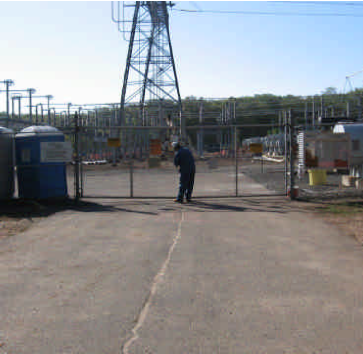
Site entrance is clean and spill kits are available onsite.
