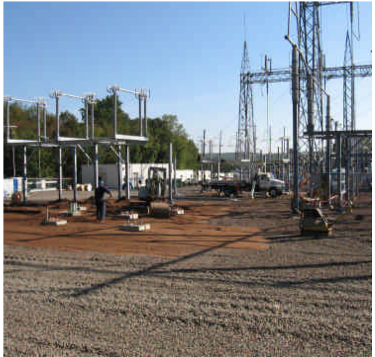
New foundations being installed in center of yard. Area is contained
