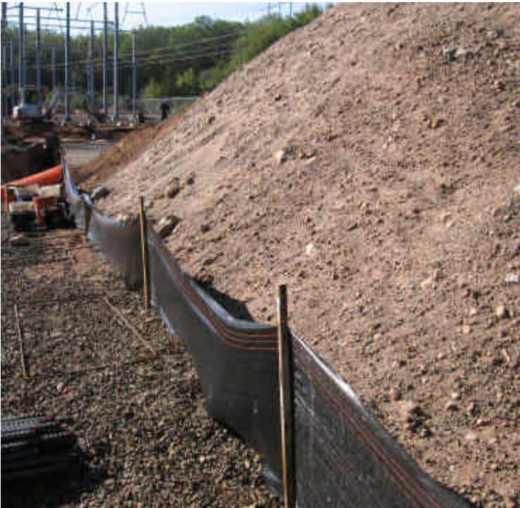
Silt fence secure in northwestern corner of site.
