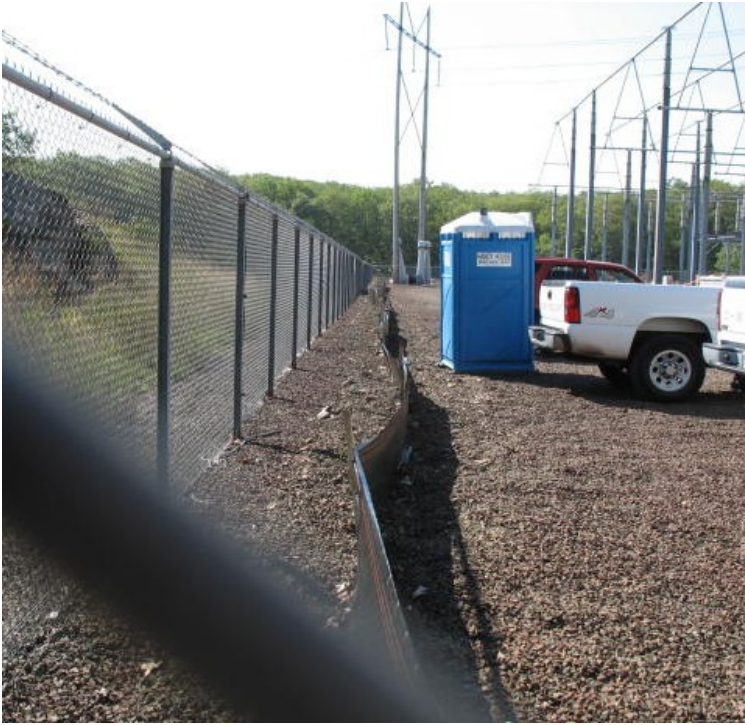
Silt fence along the eastern property looks good.
