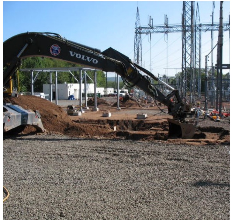
New foundations being installed in the yard. Small stockpiles remain contained.
