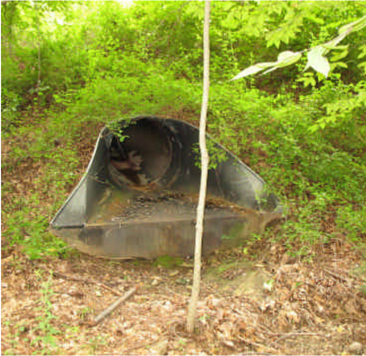
Existing culvert located under the access road to the switching station.
