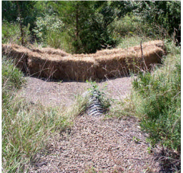
Storm water outlet pipe upgradient of the wetland, on the south side of the site. Controls are in place.
