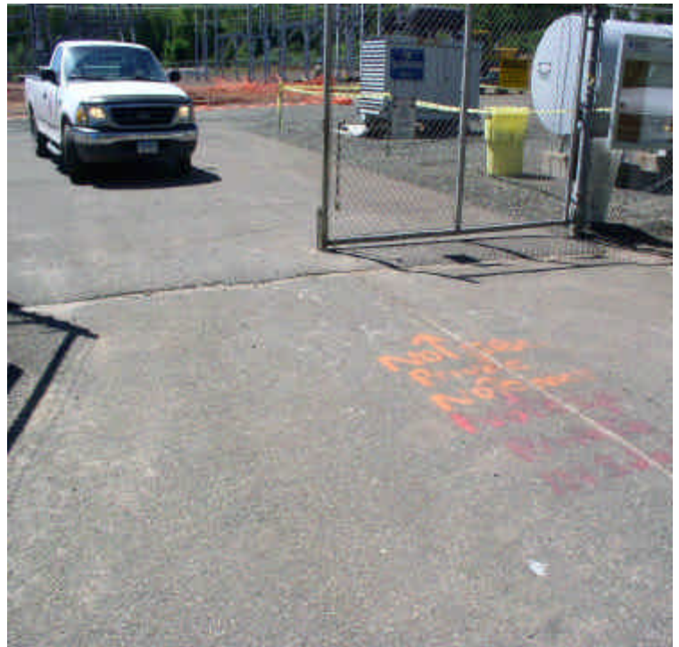
Entrance to the switching station with spill kit, north side of site.
