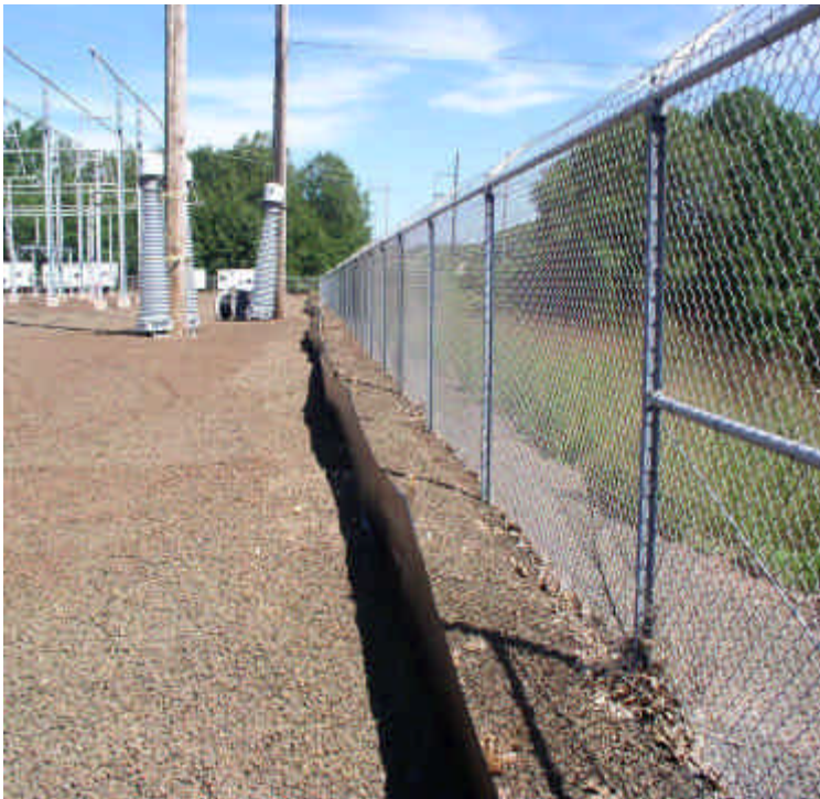
Silt fence installed along the eastern edge of the site.
