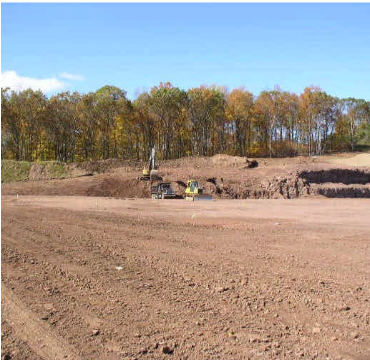
Remaining soil removal and grading along the northwestern slope.
