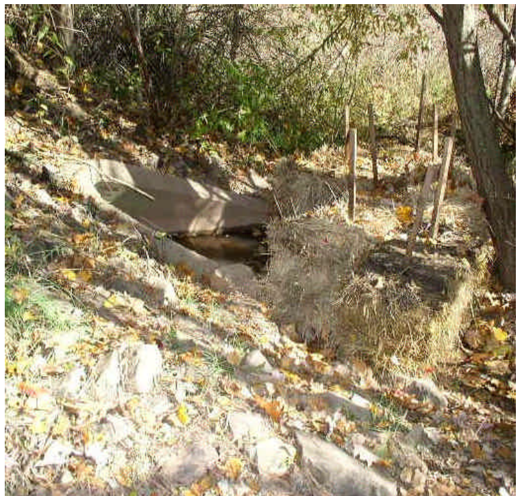
View of haybale barrier at the storm drain outlet. No new sediment has entered the wetlands.
