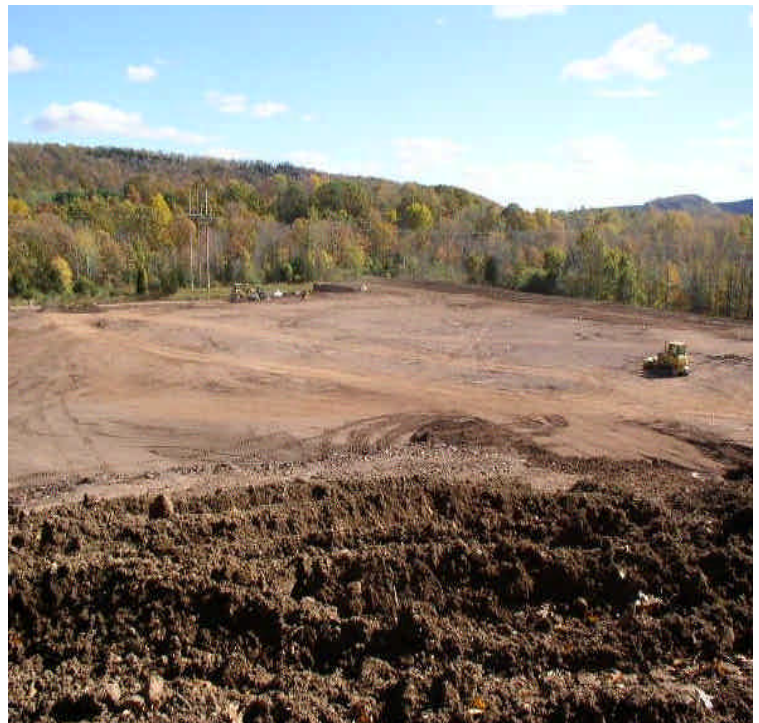
Southern portion of site, looking from northwest to southeast.
