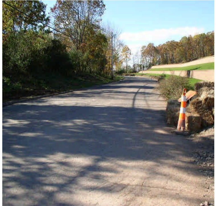
Carpenter Lane has little sediment tracking, roadway should continue to be swept regularly. The stone entrance pad was cleaned. Entrance pad improvements are planned in the near future.
