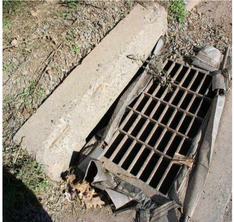
View of CB inlet protection along Carpenter Lane; dams could be placed at the curb drop inlet portion of the basin to force water through the filter.
