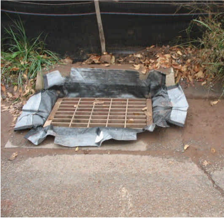
New silt liners installed in catch basins along Carpenter Lane.
