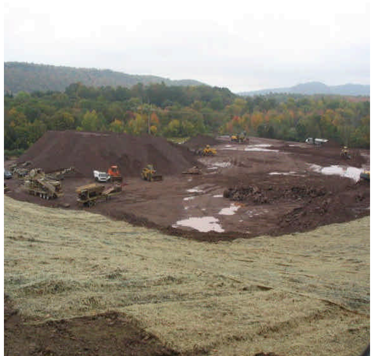
Entire site, looking from northwest to southeast.
