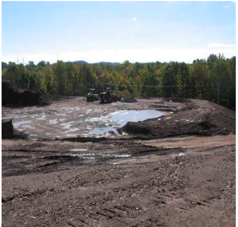
Detention pond under construction.
