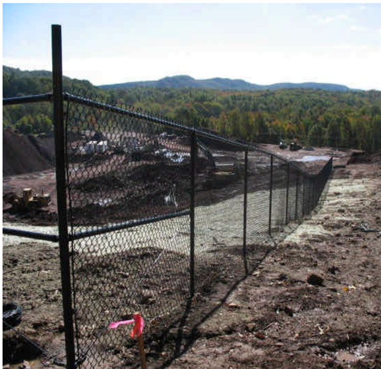
New perimeter fence installation along the western boundary of the site.
