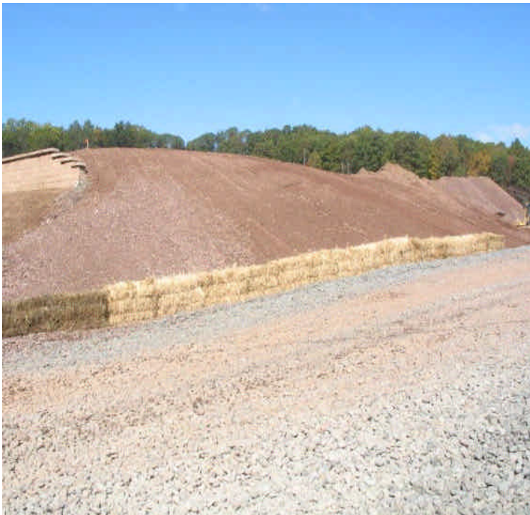
New haybales at base of detention basin slope near site entrance.
