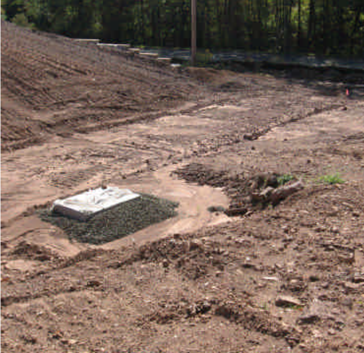
Stormwater inlet structure at southwest corner remains protected.
