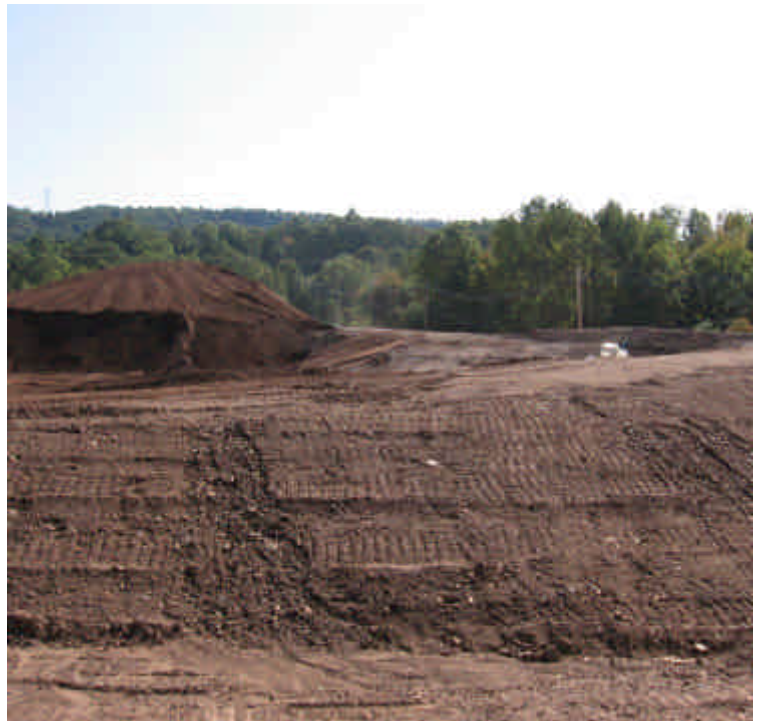
Detention pond under construction.
