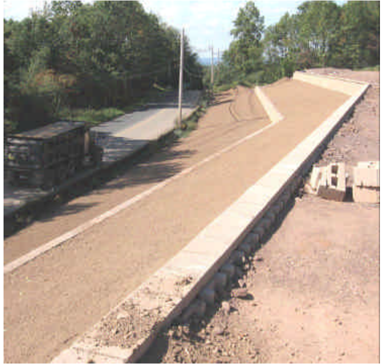
Carpenter Lane has some sediment accumulation but is being swept regularly. Southern slopes have now been seeded.
