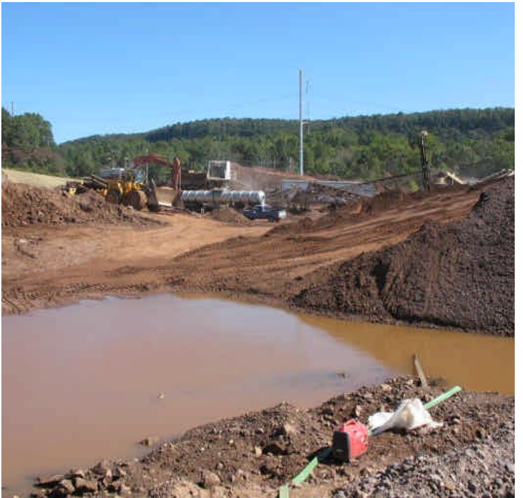
Detention pond/settling area retaining stormwater run-off.
