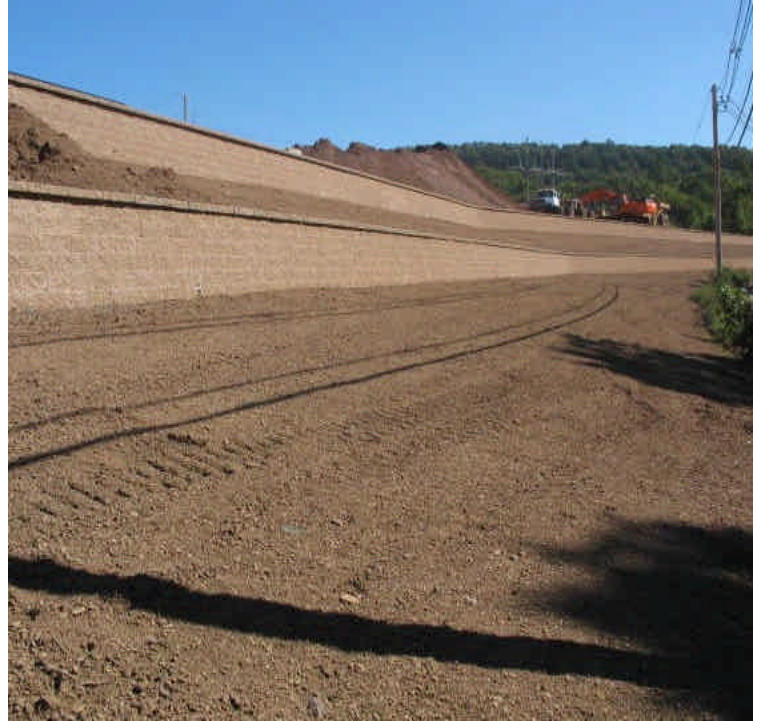
Front slopes along Carpenter Lane have been fertilized and limed, and should be hydroseeded as soon as possible. Recommended seeding time for the fall usually ends Oct 15 th .
