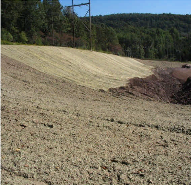
Hydroseeded northern slope with hay mat installation.
