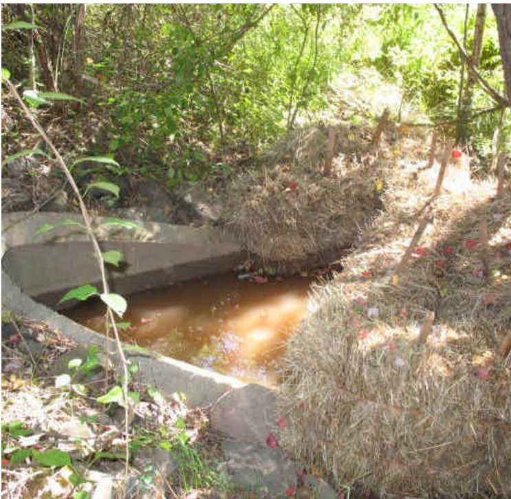
Sediment-laden water being flushed from the storm drain system and filtered before entering wetlands. Water pumping continues at night without monitoring. Sediment filled water continues to enter the wetland.
