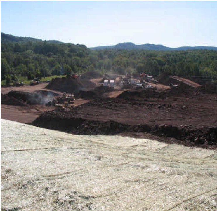
Major grading operations looking from northwest to southeast.
