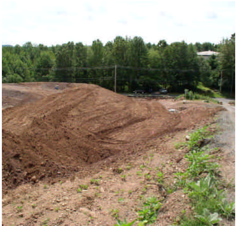
The new access driveway has been graded.
