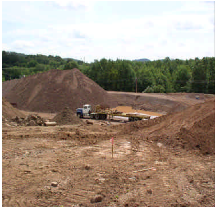
Detention pond/settling area retaining stormwater run-off. Large stockpiles are also present.
