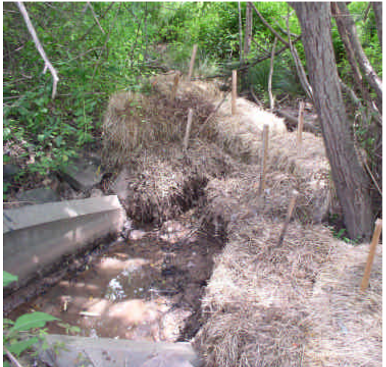
New haybales installed for additional filtration at the storm drain outlet.
