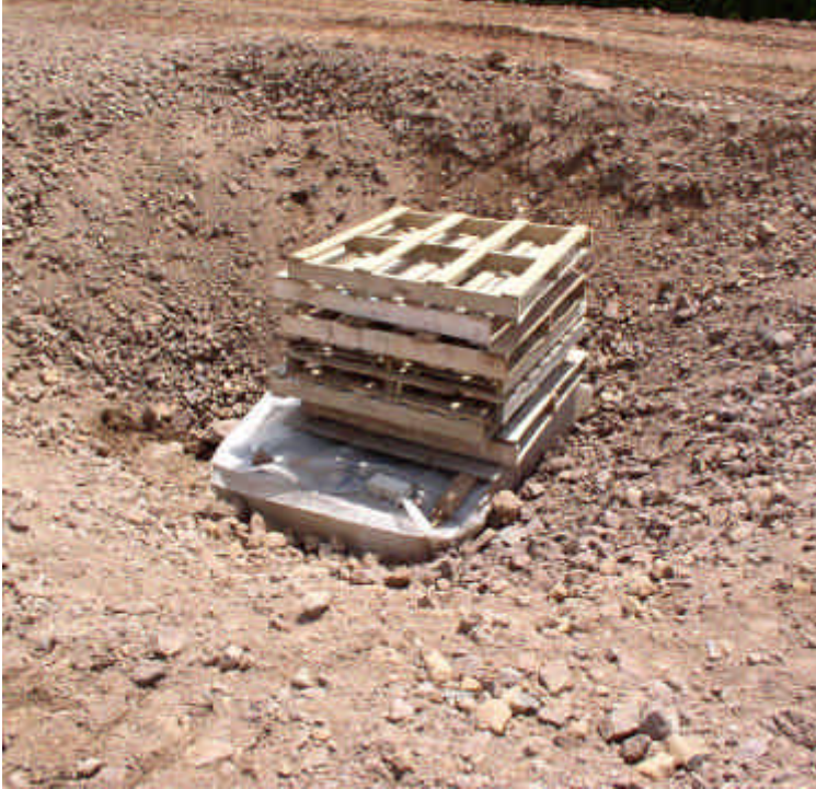
New southern catch basin, slightly raised with inlet protection.
