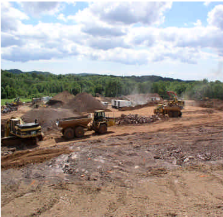
Major grading operations looking from northwest to southeast. Some airborne dust is noted. Continue to wet the soils when necessary.
