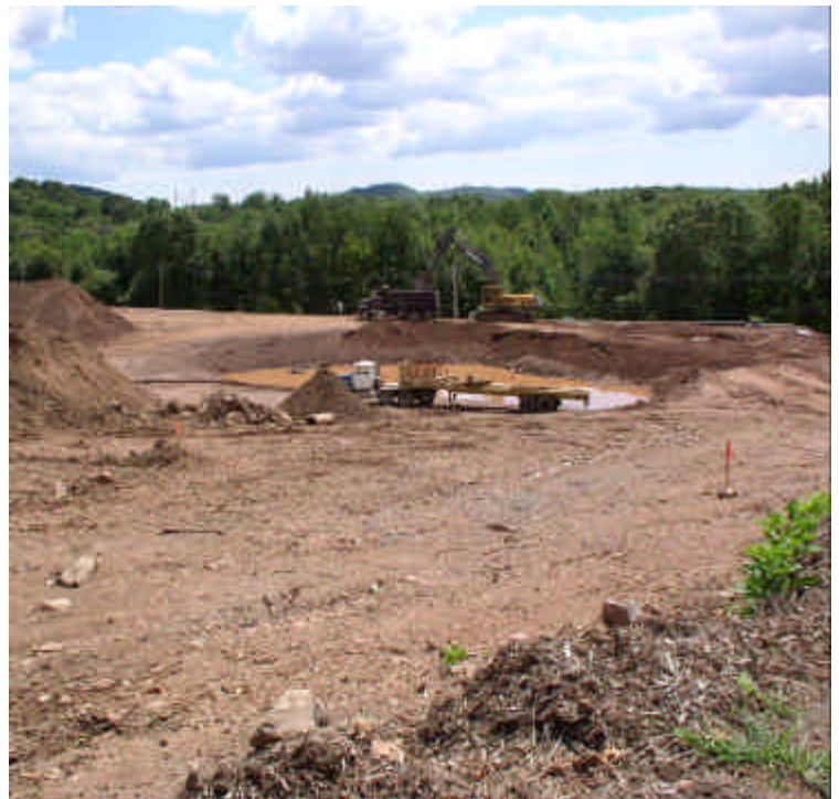
Detention pond/settling area retaining stormwater run-off.
