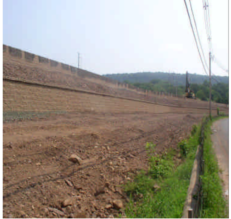
Grading and seeding remain to be done between Carpenter Lane and 1 st retaining wall.
