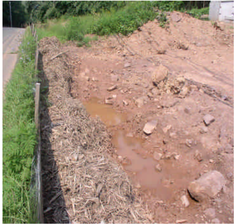
The temporary settling area in the southwest corner of the site remains in place but is holds little water at this time.
