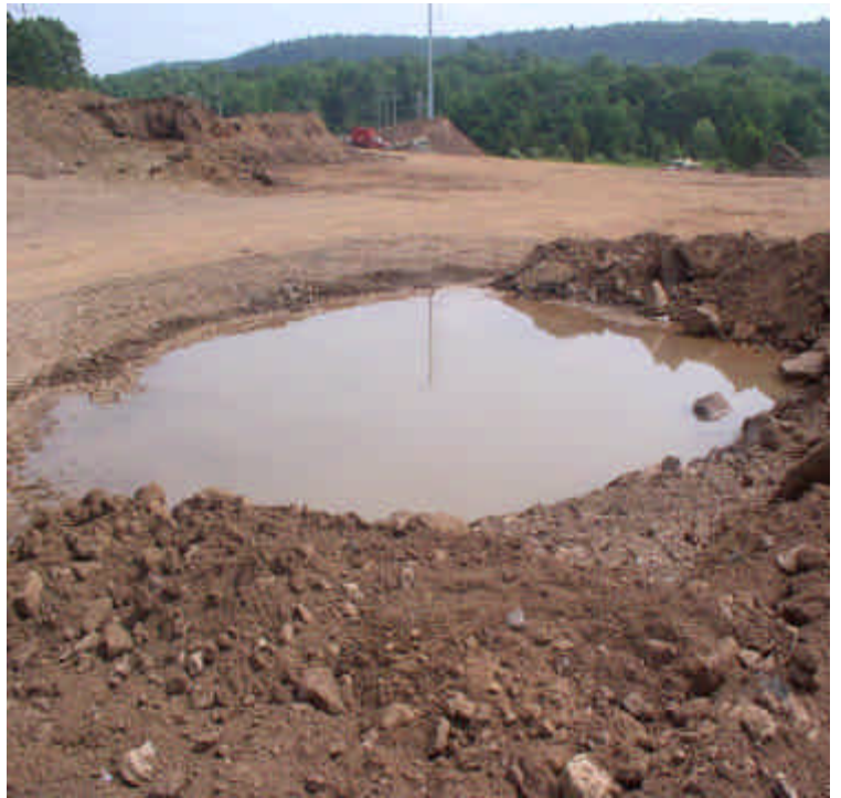
Detention pond/settling area holding pooled run-off.
