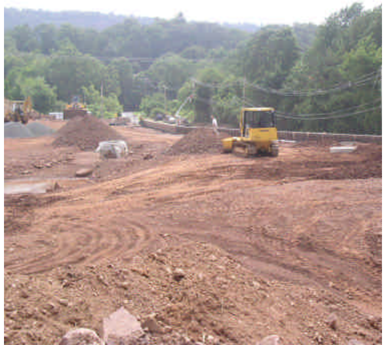
New stormwater inlet and manhole above 2 nd retaining wall.
