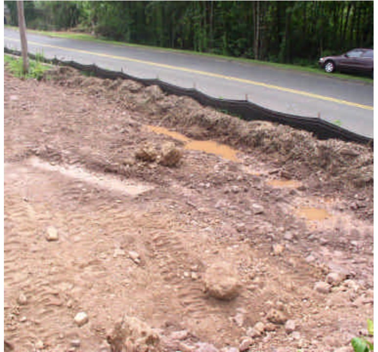
The new settling area dug in the southwest corner of the site is almost dry.
