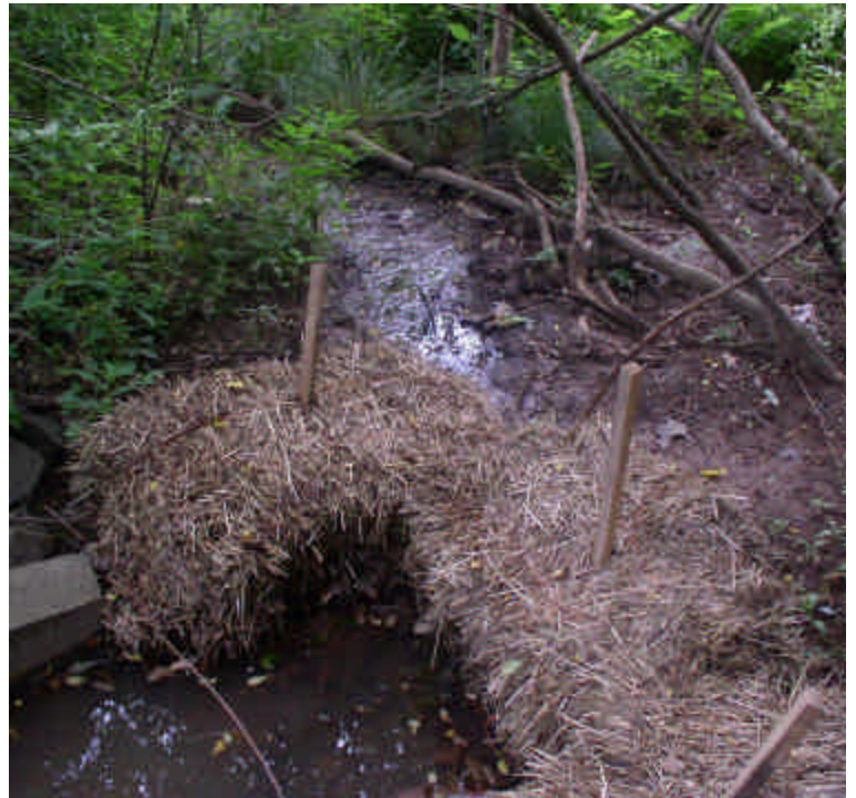
Water filtered by haybales is clearer than flow at the culvert. Sediment accumulation from the previous rain events will be removed when standing water in wetland has dried.
