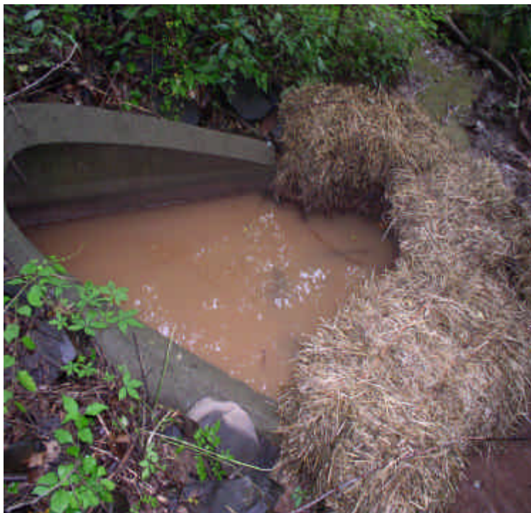
Haybales were placed for additional filtration at the storm drain outlet. Water from the outlet was still turbid.
