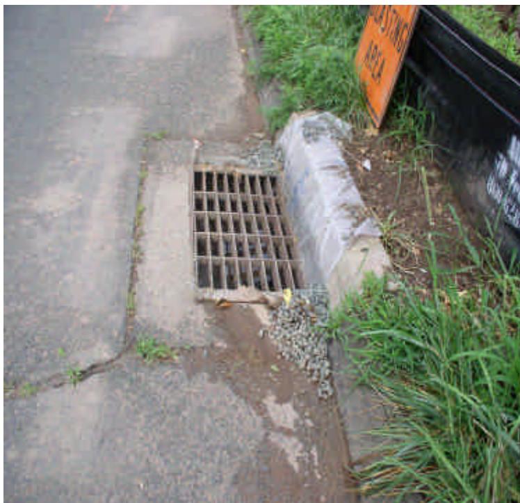
Stone in place, holding the edges of catch basin filter fabric.
