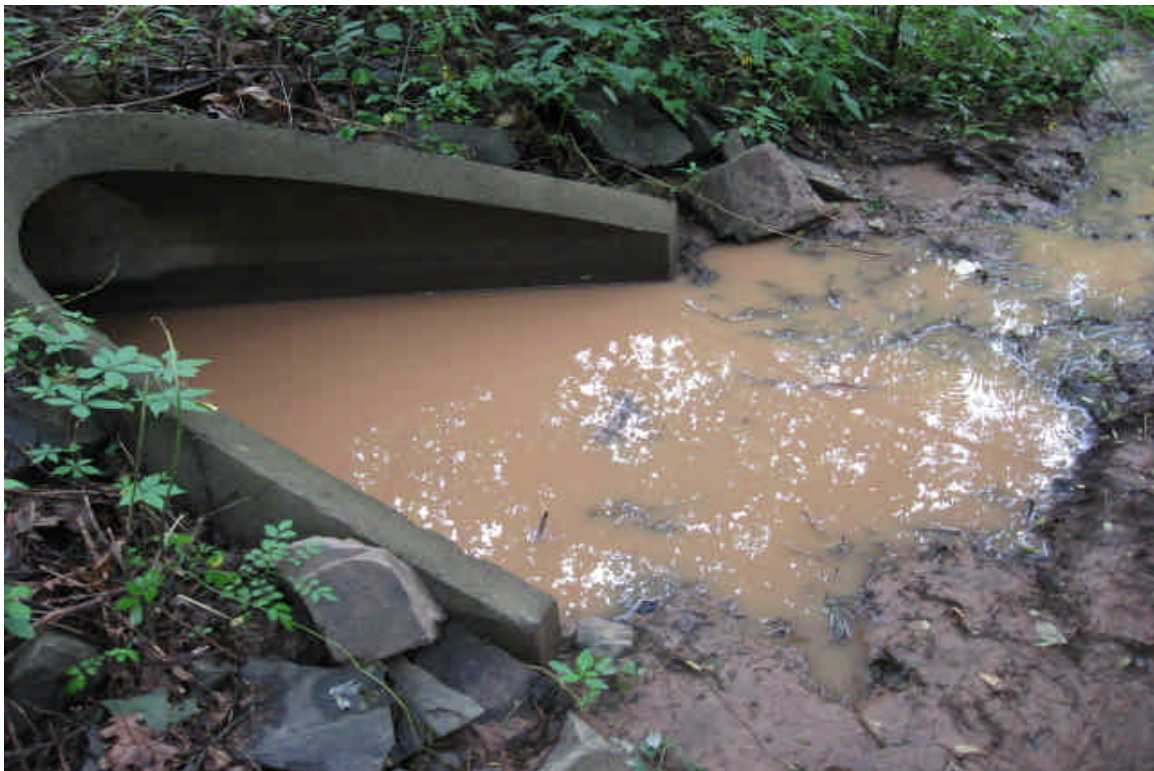
Turbid water from the site was entering the wetland across Carpenter Lane from the drain outlet after the rain event. Sediment accumulation from previous events is present here. When the area dries out, this will be removed carefully by hand.
