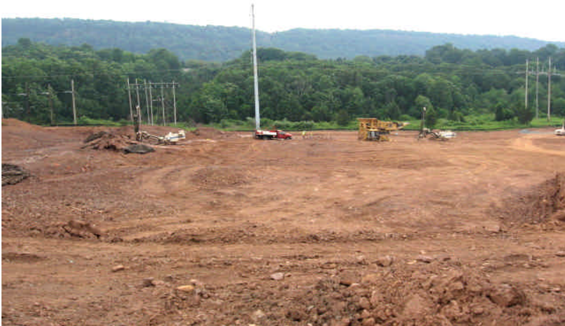
Blasting in northern part of site, viewed west to east.
