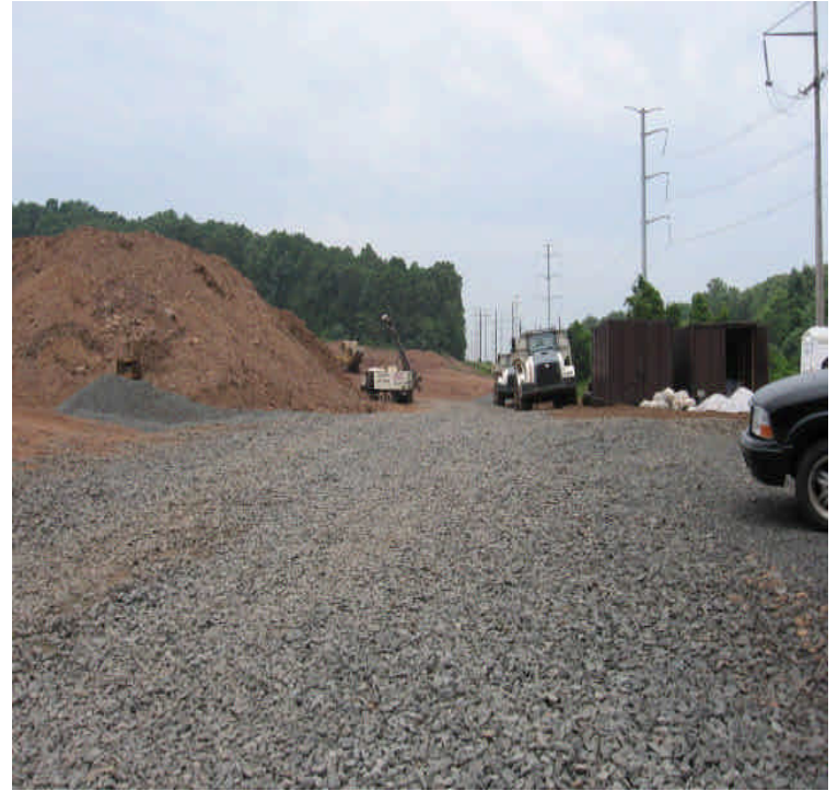
Stone construction entrance is clean.
