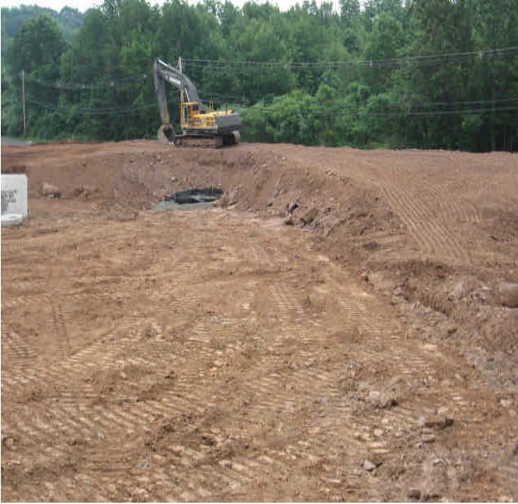
Newly constructed storm drain at south side of site.
