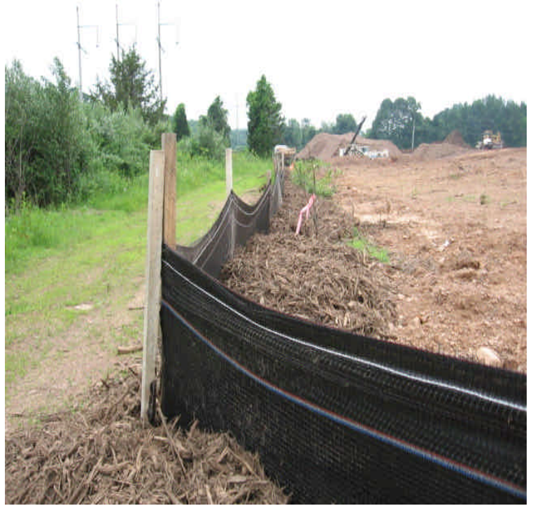
Silt fence on east side reinforced with mesh and mulch.
