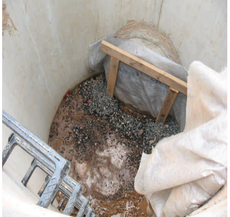
Storm drain inlet and outlet are protected with some filter fabric.
