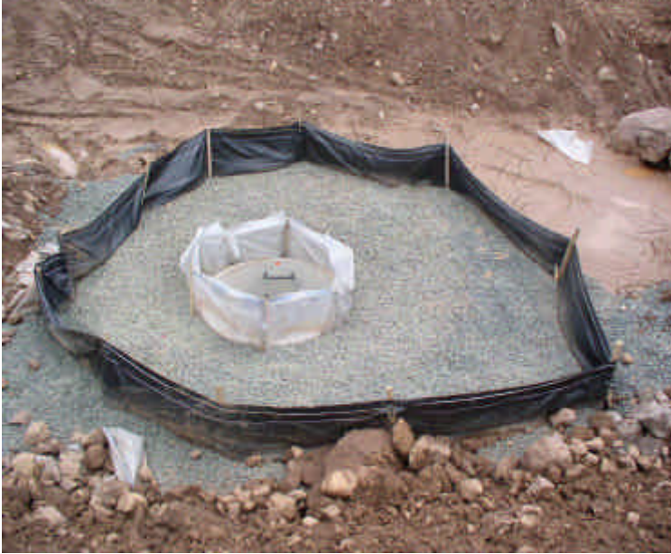
Installation of the new storm drain system with perimeter protection. Watch exposed soil around the pipe for run-off and increase controls around the pipe.
