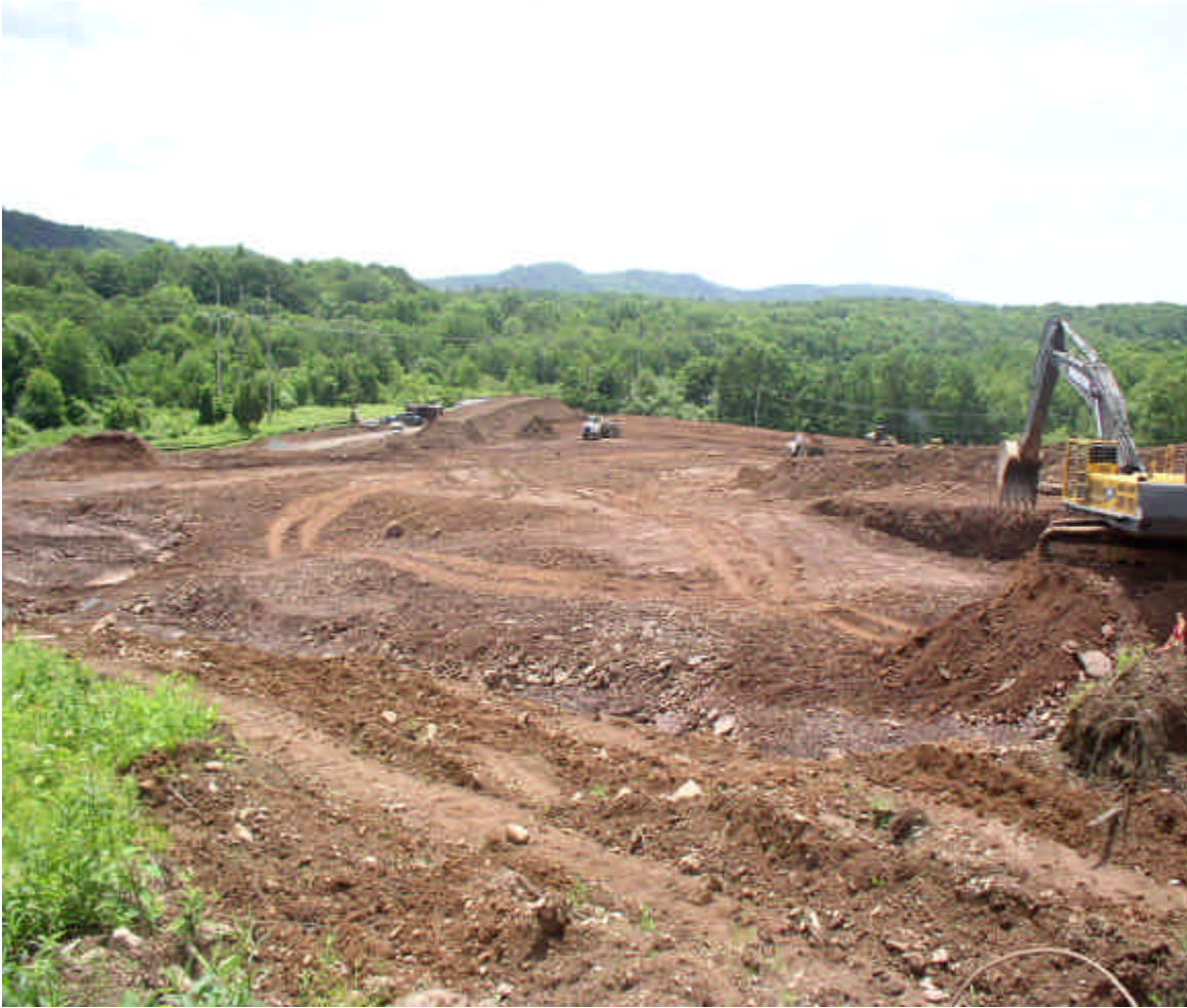
Entire site looking southeast at the major soil grading operation.
