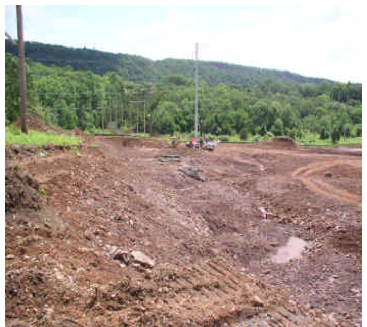
Blasting area along the north side of the site looking west.
