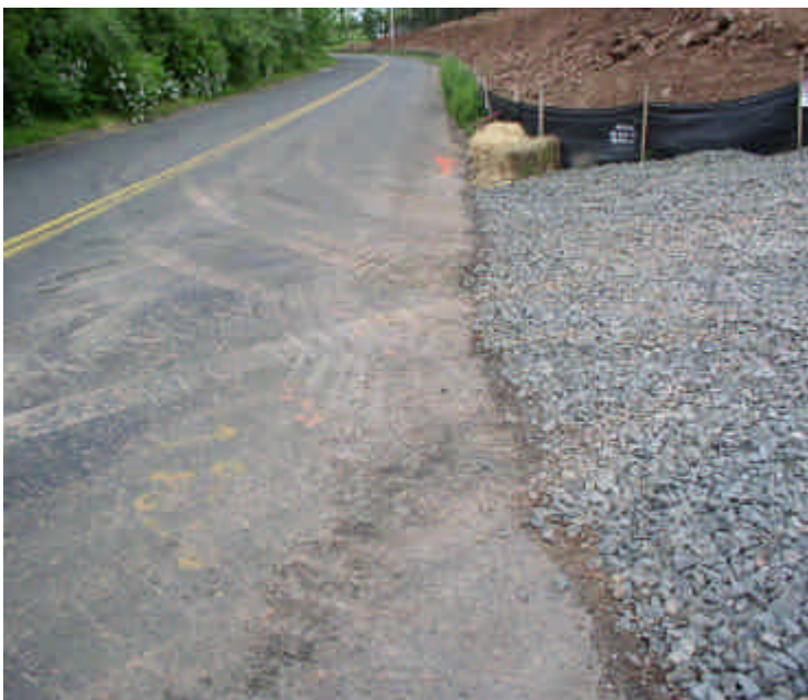
Carpenter Lane at the construction entrance.
