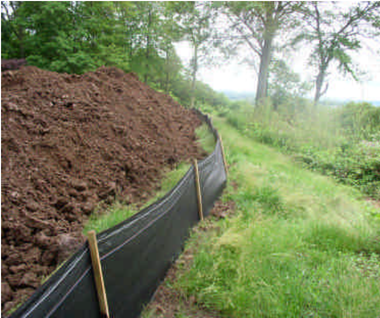
Silt fence remains in good shape around the old Zolnik property. Soil stockpiling is occurring here at this time.
