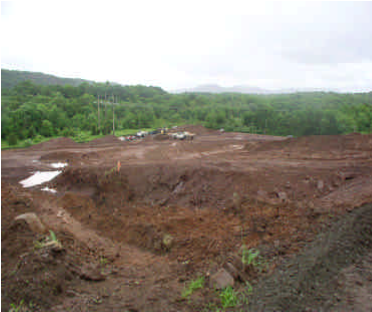
Entire site looking southeast at the major soil grading operation
