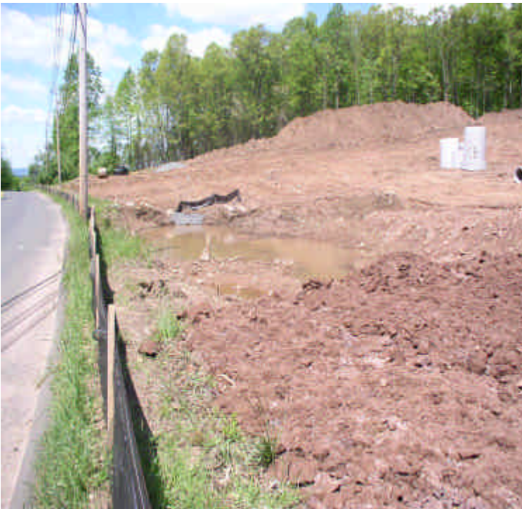
Storm water settling basin adjacent to the storm drain inlet.
