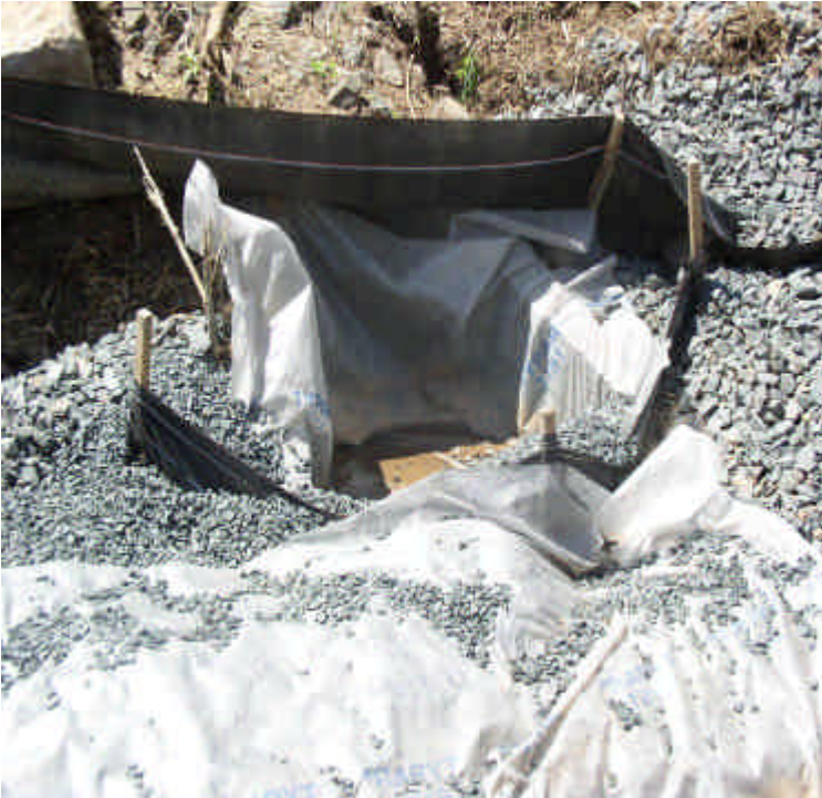
New storm drain inlet leading to wetland across Carpenter Lane. stone.
