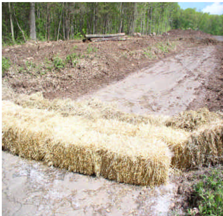
Additional haybales installed along the unused, western driveway
