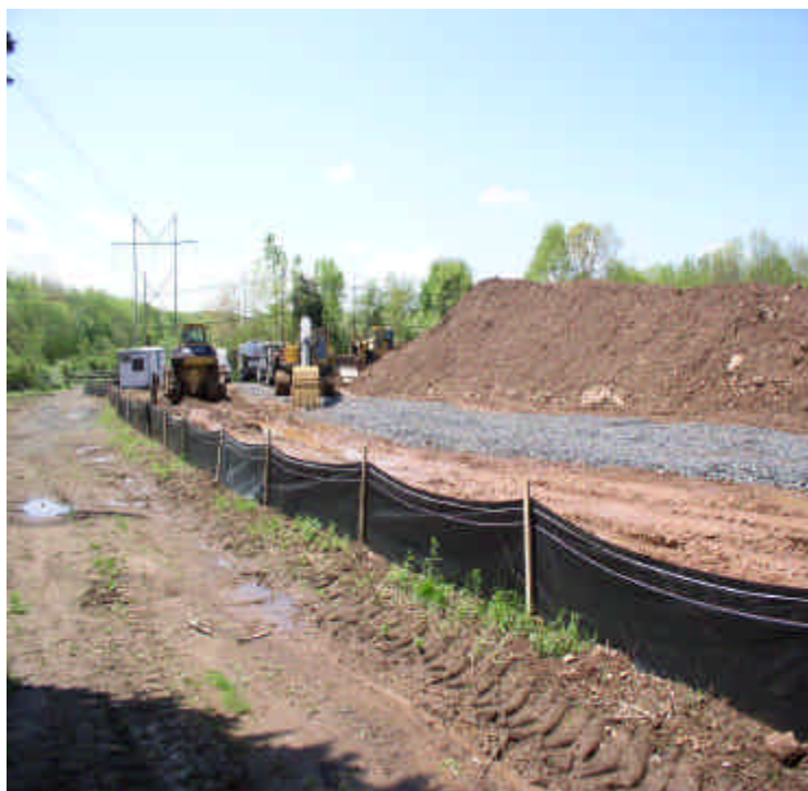
The crushed stone construction entrance was extended.
