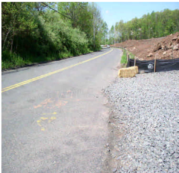
Carpenter Lane at the construction entrance. Sediment tracking was not observed.
