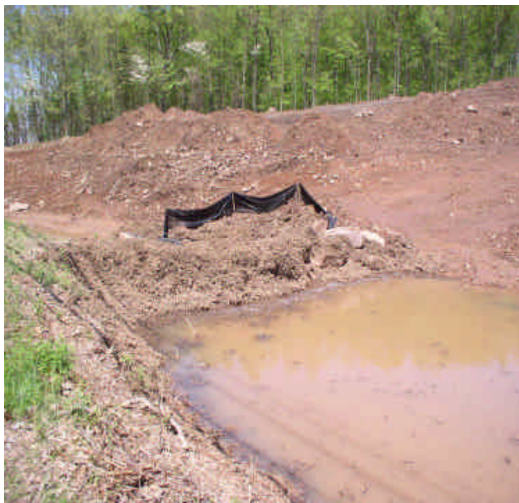
New settling basin installed adjacent to the storm drain inlet.
