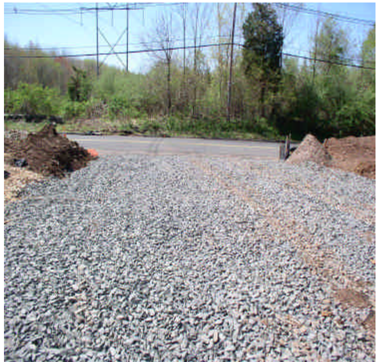
Crushed stone construction entrance at Carpenter Lane.
