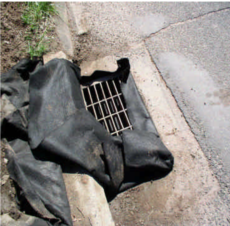
Catch basin on Carpenter Lane protected with silt sack.
