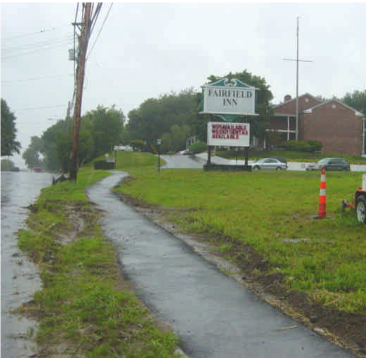
Erosion controls near vault #37 have been removed. Small amounts of exposed soil were noted as a result of removing the silt fence. Some ruts/exposed soil were also noted in the grass along the shoulder of the roadway. Mulch and seed these areas to reduce run-off.
