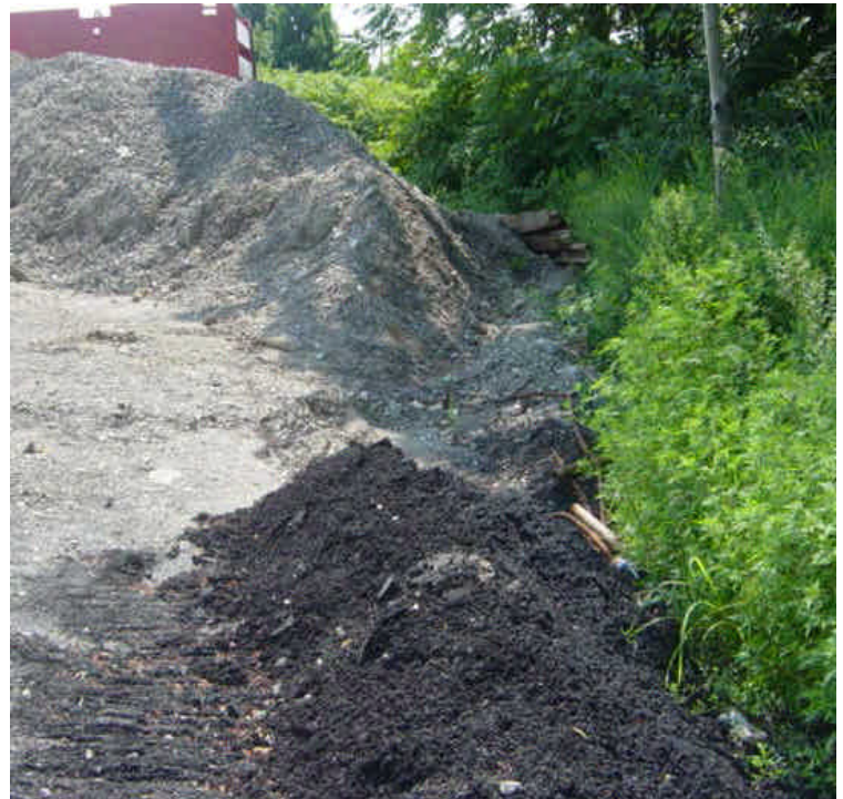
Both photos were taken within the King's Highway lay-down yard. Materials were observed overwhelming perimeter barrier controls in two locations.
