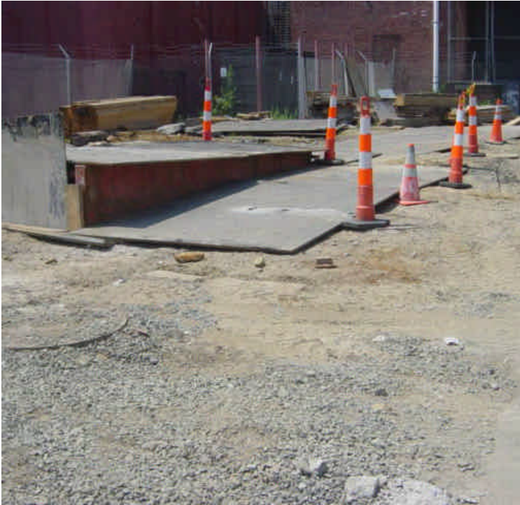
Photo of trenching activities at sta. #788 to #789.
