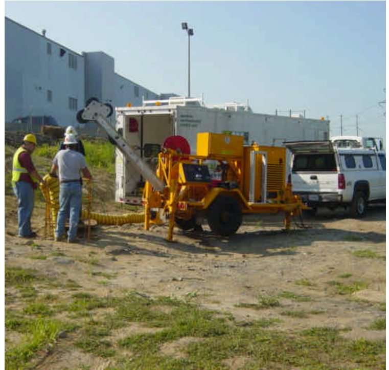
Crews were working internal to vault #5 to vault #4 during the inspection.
