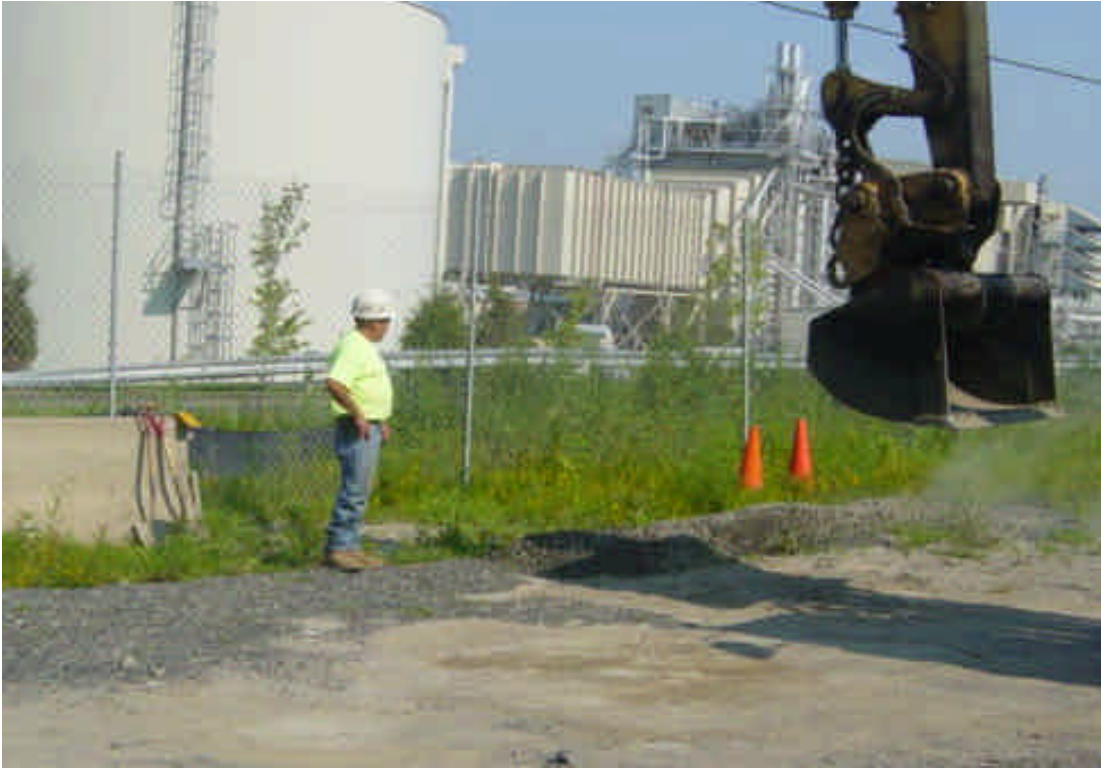
Both photos were taken within the Milford lay-down yard and are depicting a the installation of a stone berm near the entrance to the yard. The berm is being added as a barrier control to reduce sedimentation to the grassed area and the catch basin outside of the perimeter fence.
