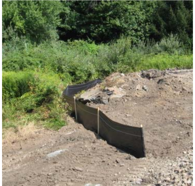
Wheelers Farms Rd: Additional silt fence is being installed as needed during pad reclamation activities.
