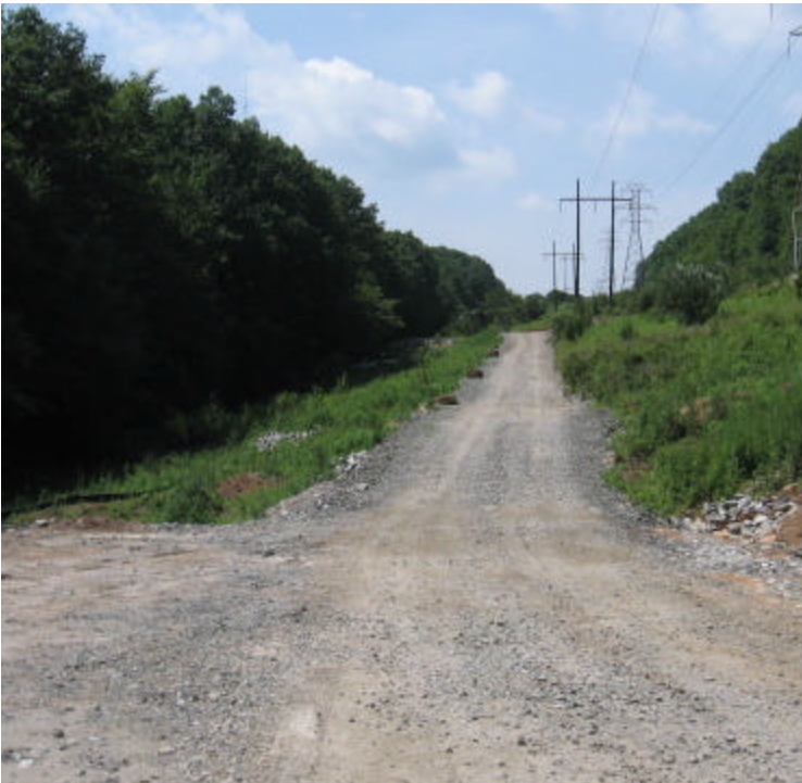
Downs Rd. (Bethany): Haybale check dams have been added at the water bar outlets for sediment filtration.
