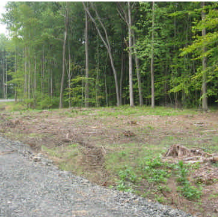
Equipment ruts were noted in a wetland west of Route 17. Continue to limit equipment to designated access roads.
