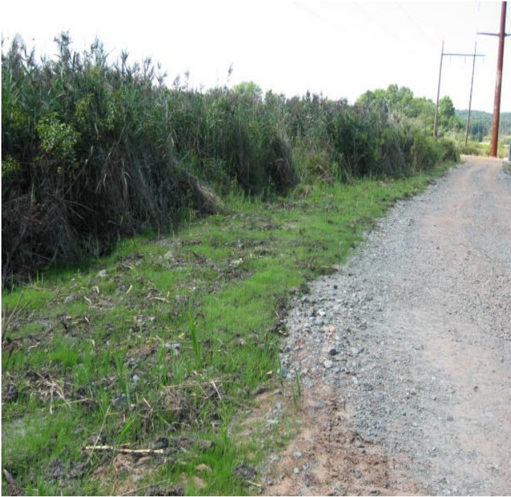
Durham Rd: Soil pile removed, disturbed areas seeded.
