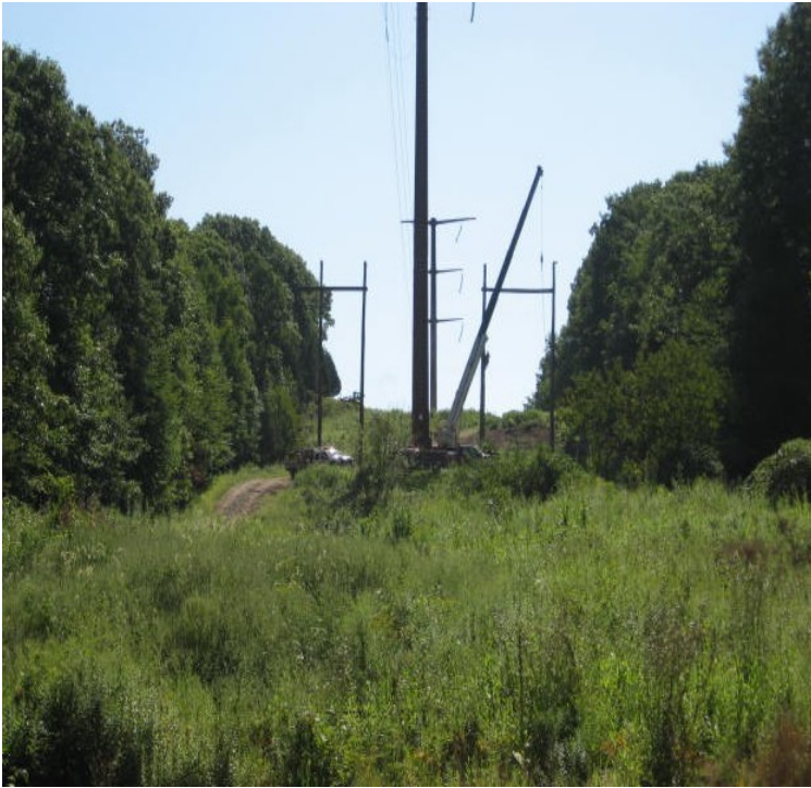
Shunpike Rd: View of pole installation.
