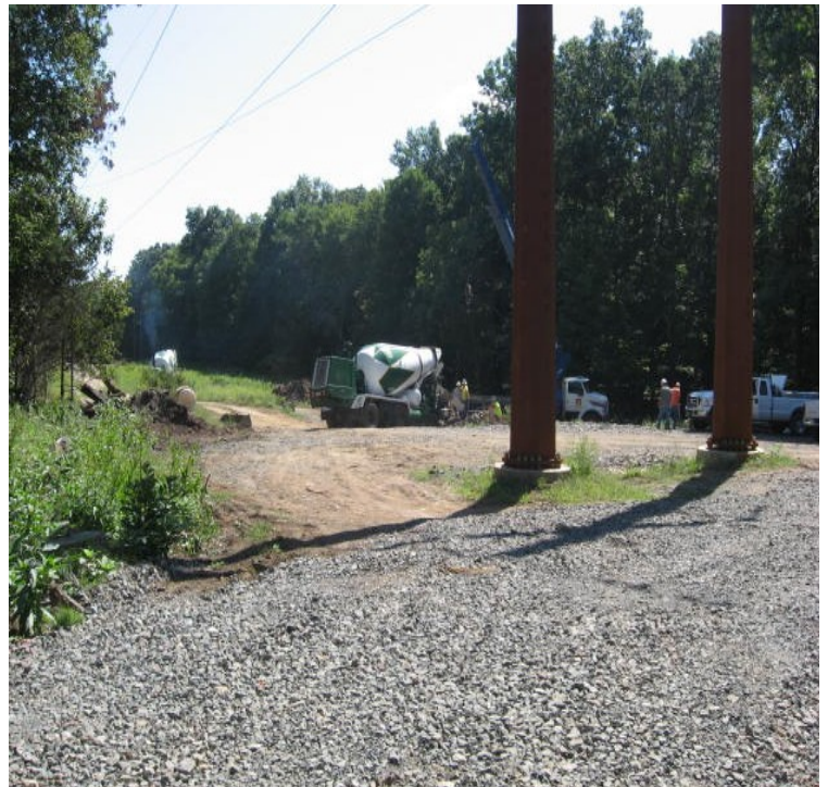
Black Walnut: Foundation pouring underway.
