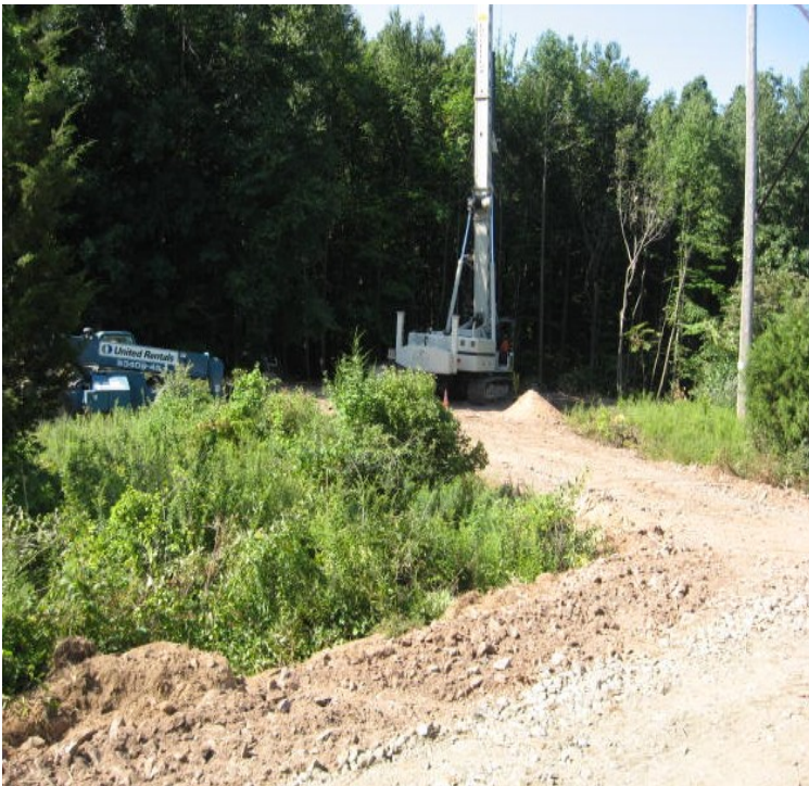
Bartholomew Rd: View of foundation drilling.
