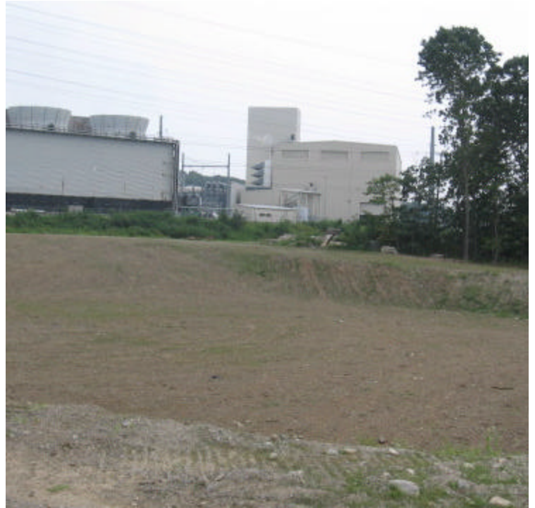
Grass growth was noted in the retention basin.
