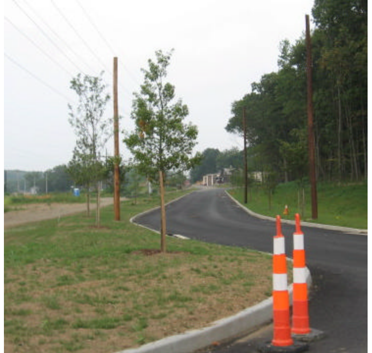
View of the recently completed Shelland Street.
