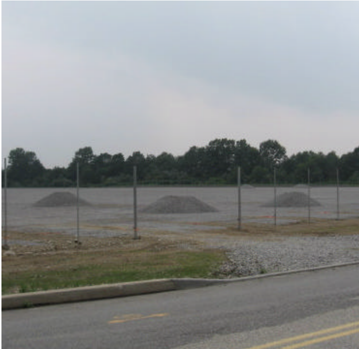
Additional gravel was delivered to the substation site this week.
