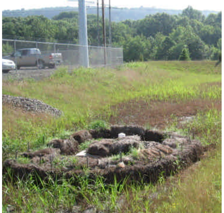
Standing water was no longer present in the detention basin. Filtering controls remain in place.
