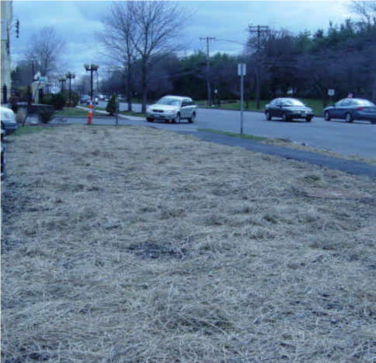
Both photo of temporary stabilization measures (mulch) on exposed soils at completed vault locations. Left: Vault #20. Right: Vault #23.
