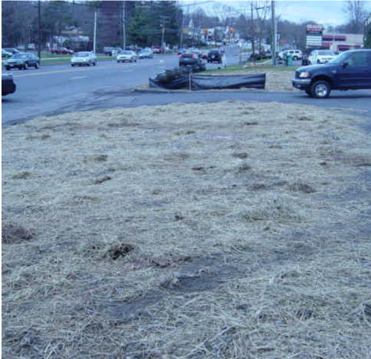
Both photo of temporary stabilization measures (mulch) on exposed soils at completed vault locations. Left: Vault #20. Right: Vault #23.
