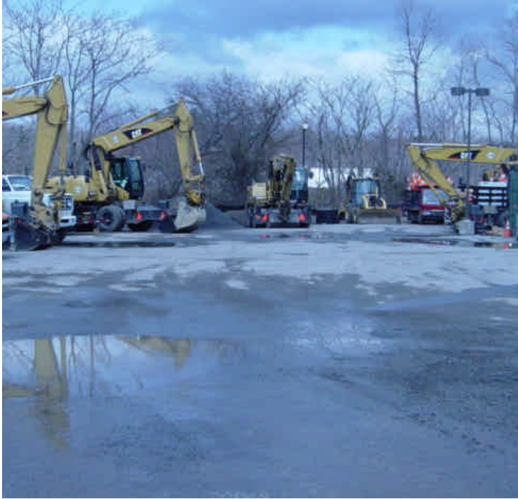
Photo of the Imperial Ave. lay-down yard. No issues were noted.
