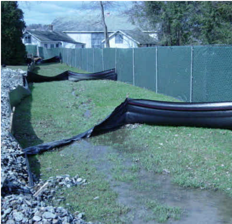
Both photo taken within the Sherwood Island lay-down yard. Left: Silt fence check dam leading to stormwater outlet has been compromised and is in need of repair. Right: Fluid filled equipment being stored on grassed area. No leaks were observed but equipment could be stored on a liner or otherwise contained proactively.
