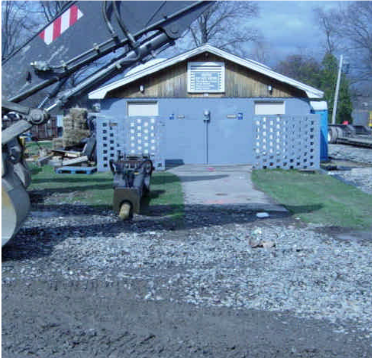
Both photo taken within the Sherwood Island lay-down yard. Left: Silt fence check dam leading to stormwater outlet has been compromised and is in need of repair. Right: Fluid filled equipment being stored on grassed area. No leaks were observed but equipment could be stored on a liner or otherwise contained proactively.
