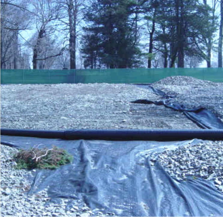
Both photos show the Sherwood Island lay-down yard. Left: View of an area in the process of being set-up for use by the contractors. The area is lined with fabric and a mixture of stone/soil is applied. Another layer of fabric is placed, and finally the area is covered with stone. Right: Good erosion controls are in place to protect the only stormwater outlet from the site. The section of silt fence in the foreground of the photo is in need of repair.
