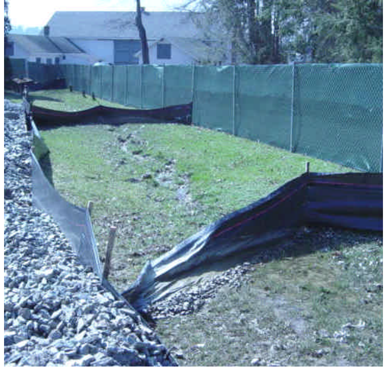
Both photos show the Sherwood Island lay-down yard. Left: View of an area in the process of being set-up for use by the contractors. The area is lined with fabric and a mixture of stone/soil is applied. Another layer of fabric is placed, and finally the area is covered with stone. Right: Good erosion controls are in place to protect the only stormwater outlet from the site. The section of silt fence in the foreground of the photo is in need of repair.
