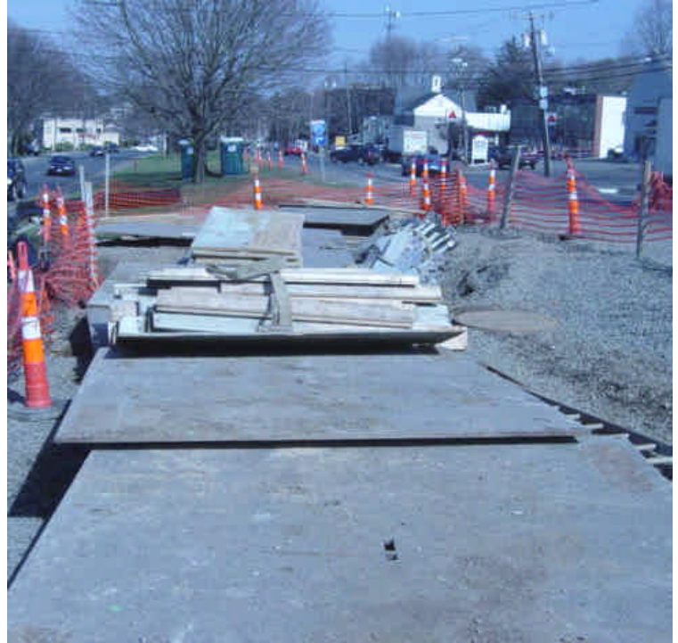
Photo of vault #18 construction activities.
