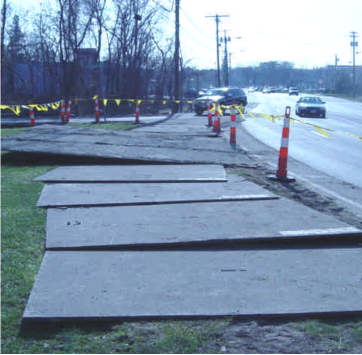
Both photos are of trenching activities at sta. #608 to #609. Right: A small amount of bituminous concrete has been piled along the edge of the trench work/roadway. When feasible, remove the excess construction materials/debris from the site.
